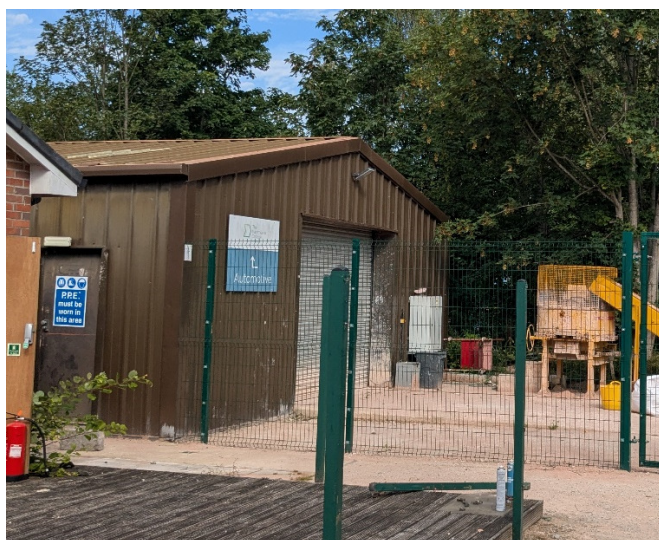
Existing Brick Workshop
