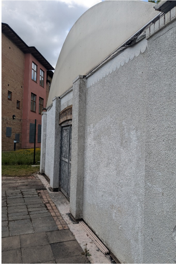
Existing polytunnel building
