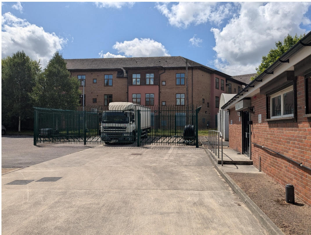
Existing secure compound for HGVs. Bungalow building is visible to the right-hand side.
