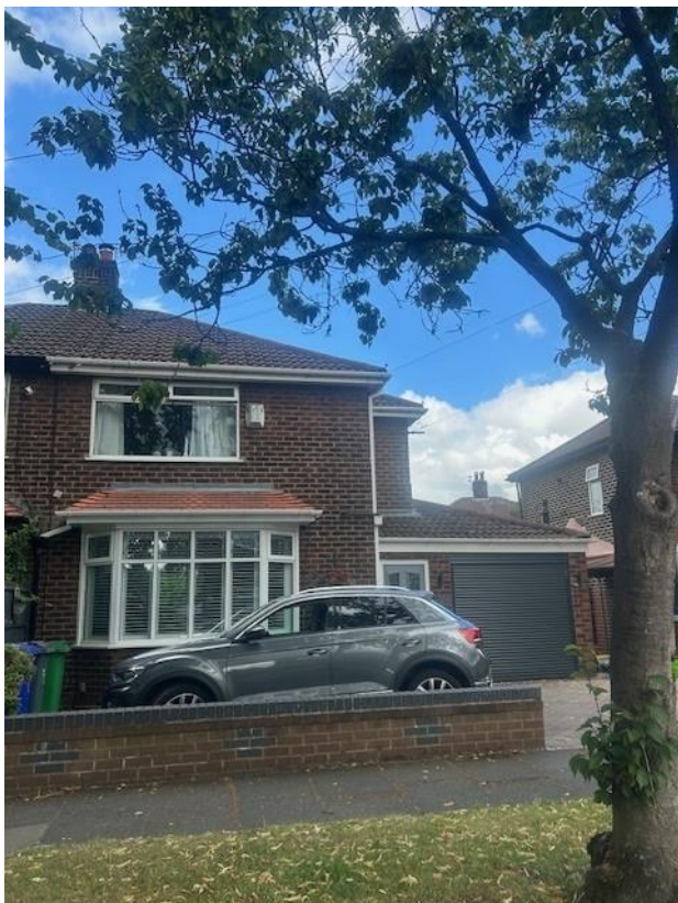
Figure 1, Front elevation of 32 Penarth Road.
