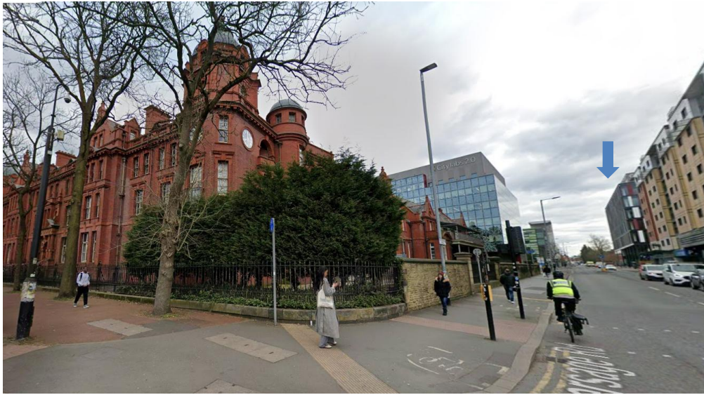
Figure 14 – A view looking east into Hathersage Road from Oxford Road, showing the Grade II Listed St Mary's Hospital holding the corner of the two streets to the left, and the Citylabs 4.0 building (marked by arrow to the right). The sites of the proposed gas stores are located behind the buildings to the right (Source: Google)
