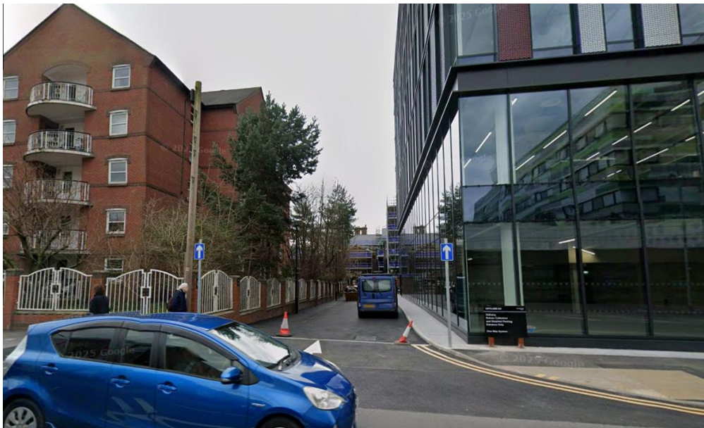
Figure 13 – A view looking south into the eastern vehicular access road from Hathersage Road, showing the newly completed Citylabs 4.0 building (right) and the ongoing construction of the St Gabriel's development to the southern end of the drive. (Source: Google)
