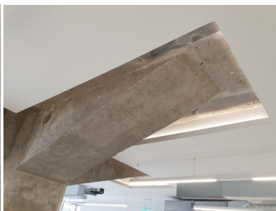
Image 6: Underside of cruciform concrete column
