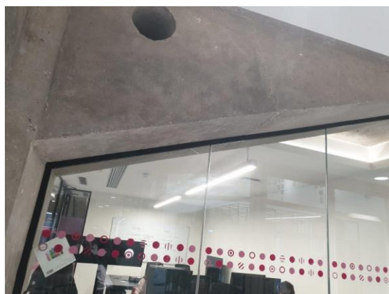
Image 10: Ground floor. Glazed partition abutment.
