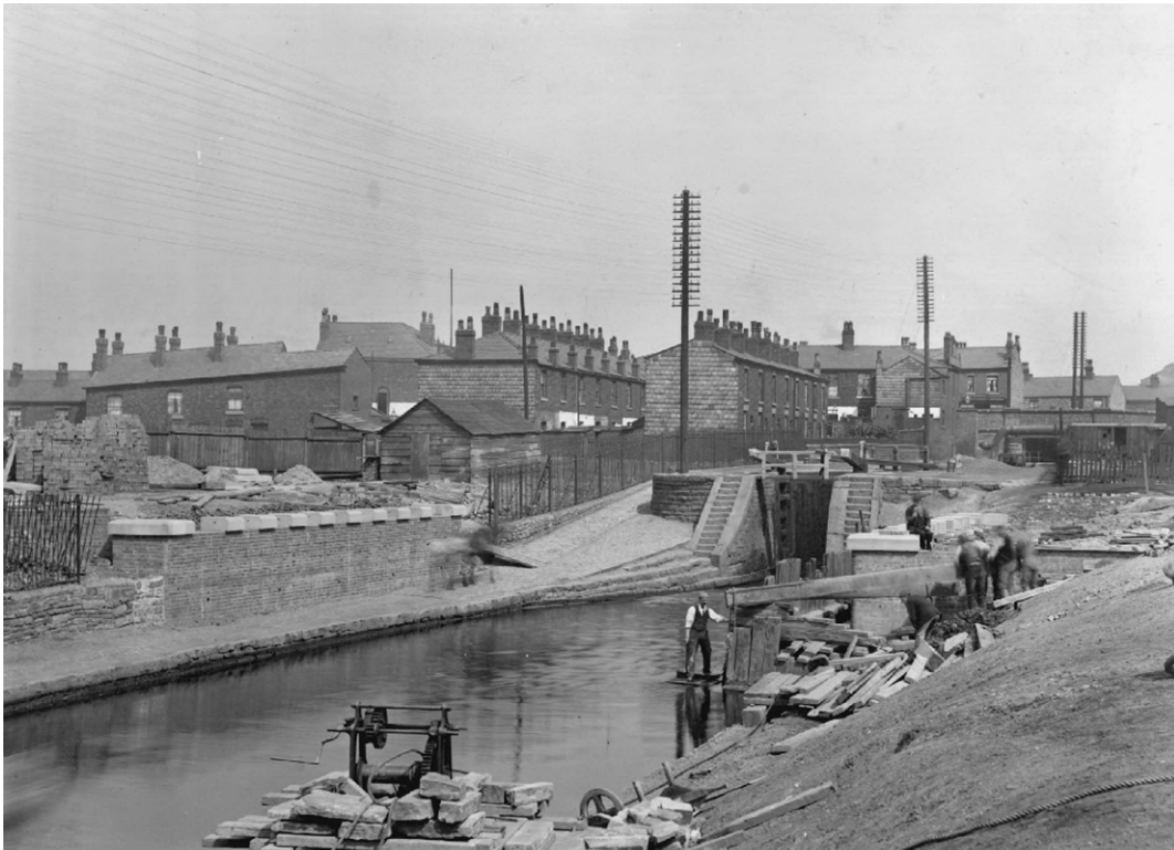
Figure 5. Forge Lane site for bridge over Canal (A Bradburn, 1903). Photo taken looking north east, with Canal Lock 6 visible at the centre of the image, and Mill Street bridge to the far right. The Site is located to the far side of the canal, just out of shot to the left of the frame.
