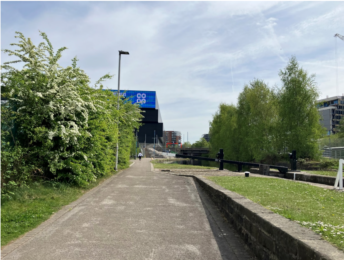
Figure 21 Looking east along Ashton Canal (Source: Planit, 2025). Proposed development shown as red wireline
