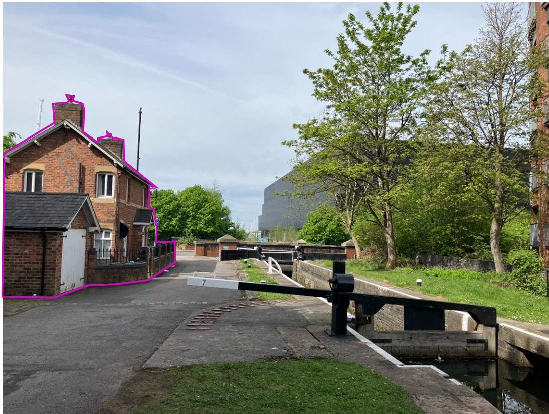
Figure 17 Ashton Canal Lock Keepers Cottage on South Side of Lock Number 7 of Ashton Canal (Source: Authors own, April 2025) Asset outlined in pink
