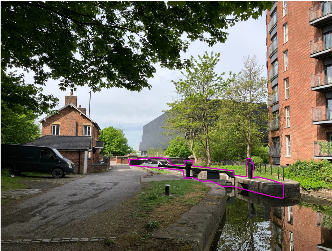
Figure 16 Ashton Canal Lock Number 7 with Roving Bridge Immediately East of Mill Street Bridge (Source, Authors Own, April 2025) Asset outlined in pink
