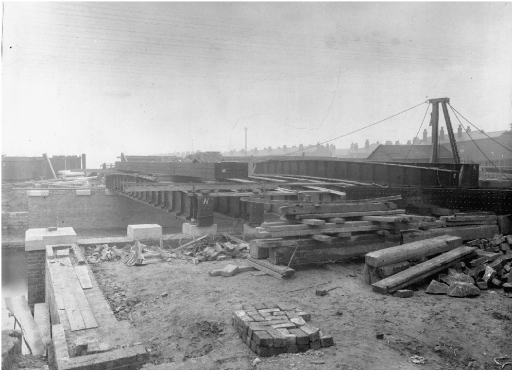
Figure 6 Forge Lane bridge under construction (A Bradburn, 1903). Photo taken looking north, the Site located just out of frame to the left.
