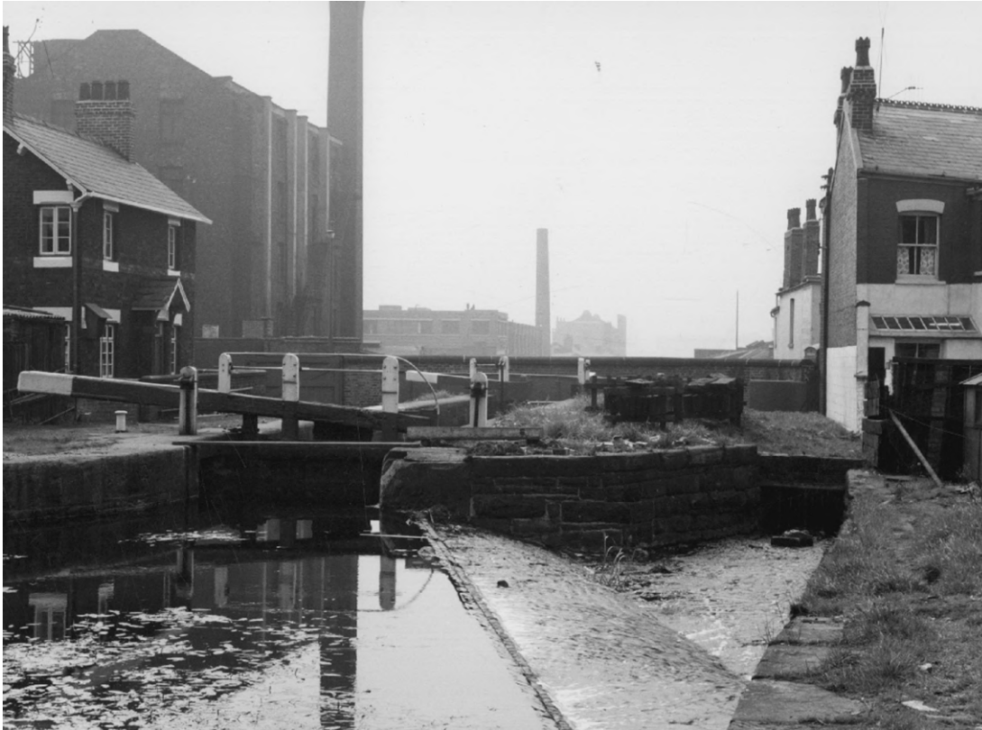
Figure 10 Ashton-under-Lyne Canal: 141, Manchester, Mill Street Bridge (L Kaye, 1960). Looking west toward Mill Street Bridge, with Lock leepers cottage to left side of frame, and Lock 7 in the foreground. The Site is located in background, beyond Mill Street bridge.
