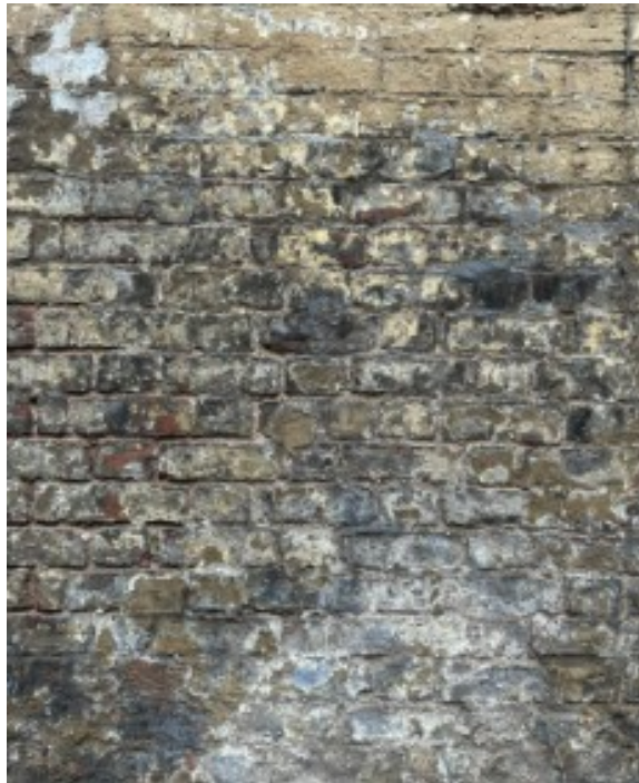
Courtyard brickwork before cleaning
