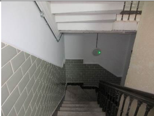
Light to stair turn between ground and 1 st
