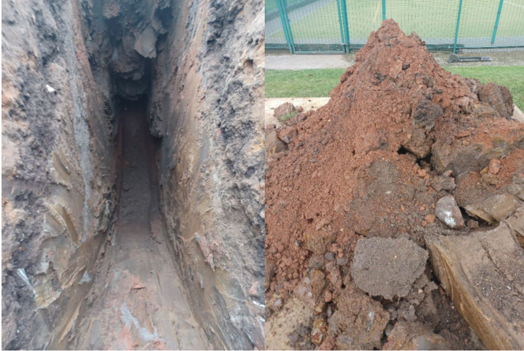
TP02 – Excavation and view of arisings
