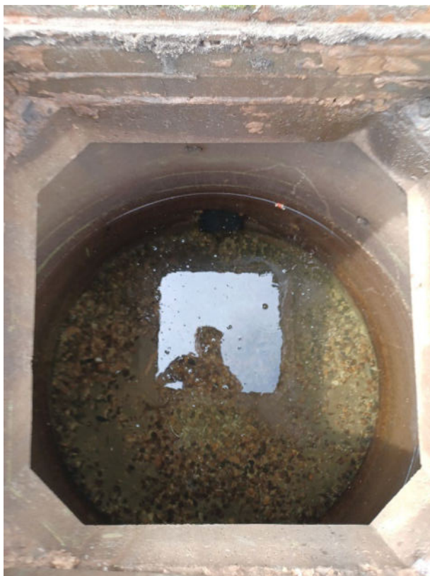
Photograph 2.2.4 Inside the existing presumed soakaway chamber adjacent to the south east corner of the pitch, showing standing water within.
