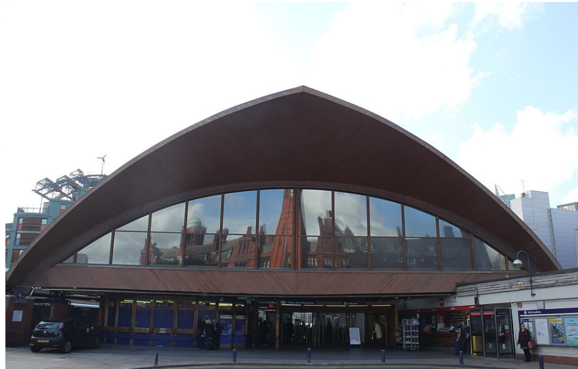
Grade II listed timber façade of the station.
