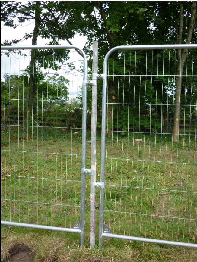
Tree Protective Fencing Specification
