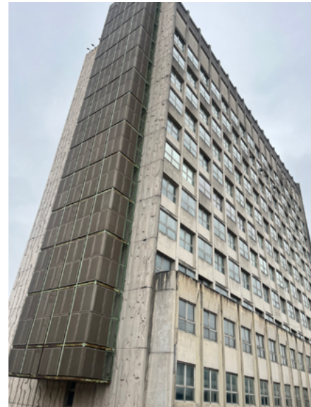
Top left image: North-West building corner with glazed western elevation, sculpted concrete panels and metal cage-style encasement to plant equipment.
