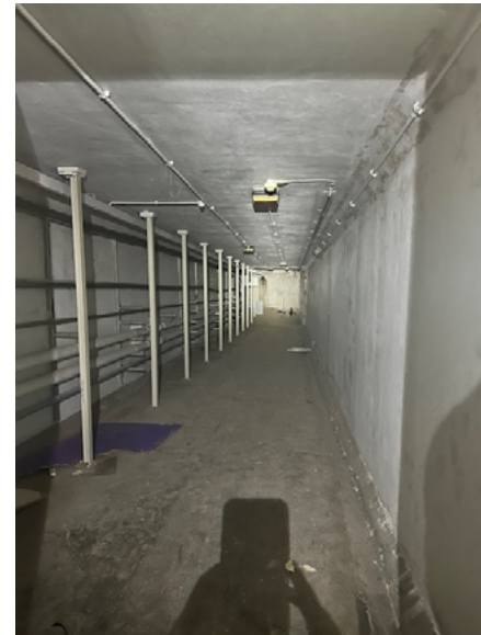
Image: View through tunnel looking East, towards Masdar Building
