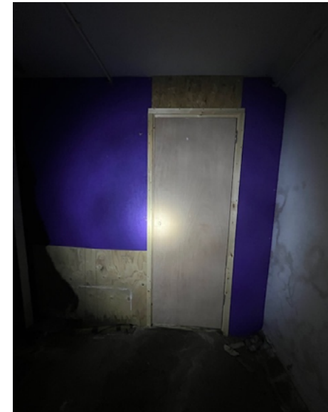
Image: View through tunnel looking West, to temporary hoarding within the Faraday Basement
