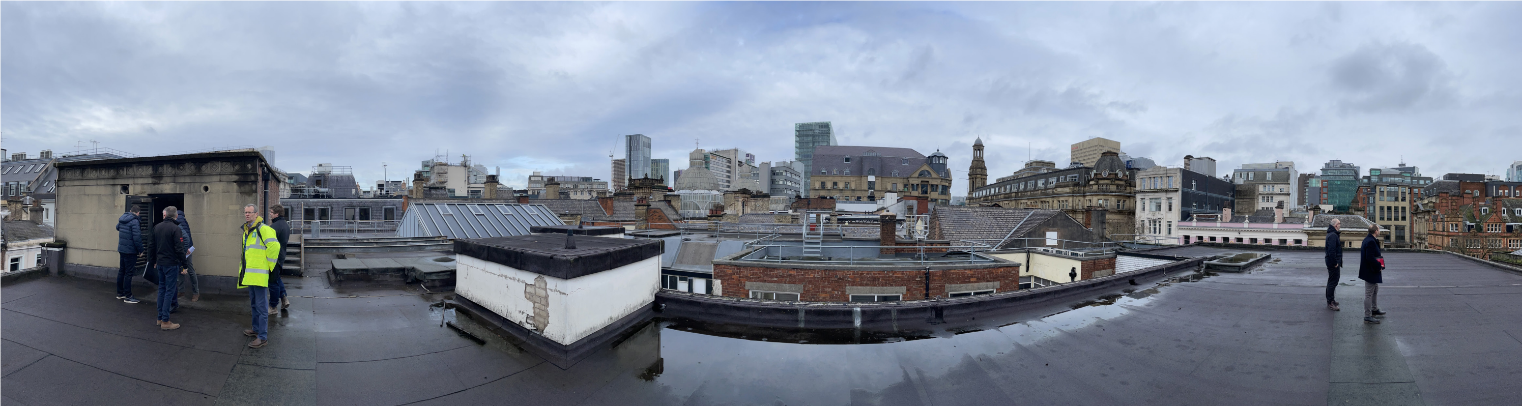
Panorama View to North - Secondary
