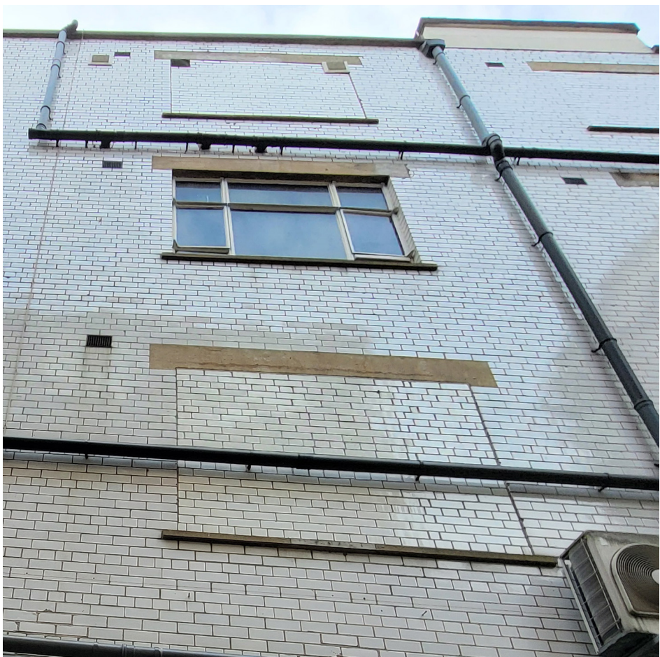
Typical Courtyard North Elevation Bay - Existing Site Photograph
