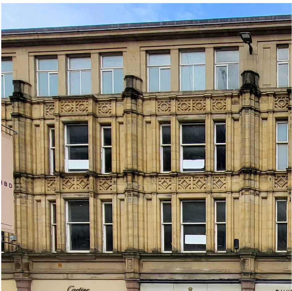
Typical Street Facing South Elevation Bay - Existing Site Photograph
