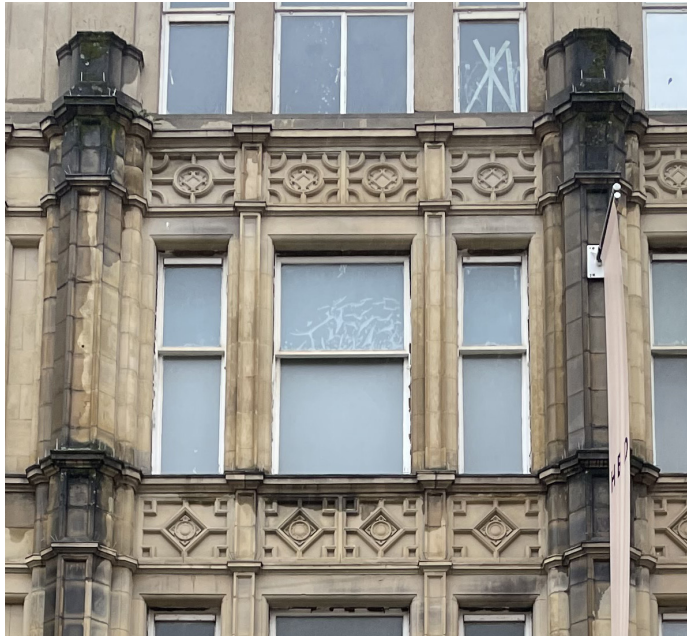
Typical Bay with Masonry Detailing (horizontal & vertical)
