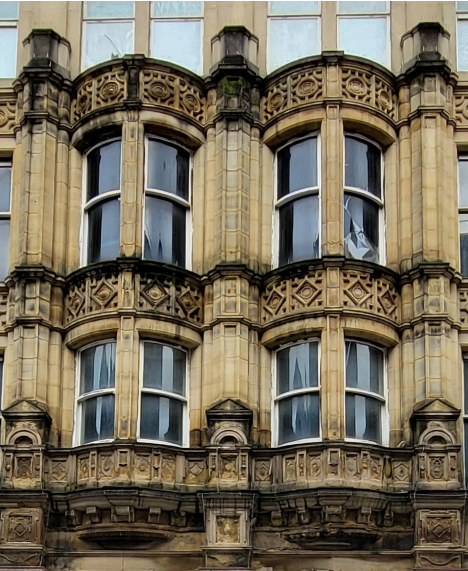
Oriel Window & Masonry Detailing (horizontal & vertical)
