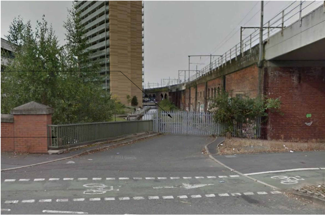
Existing Site Entrance
