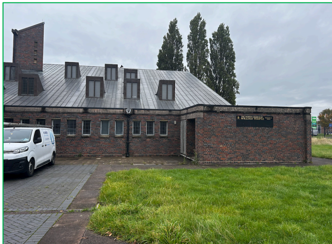
u1b5/6 Developed land; sealed surface of the building and access
