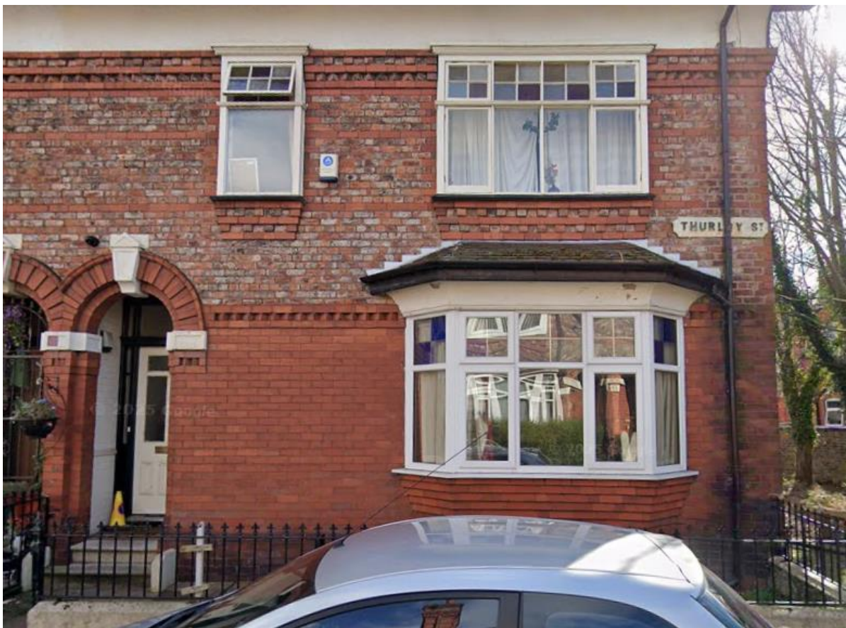
Figure 1. Front Elevation, Google Street View June 2024, accessed September 2025
