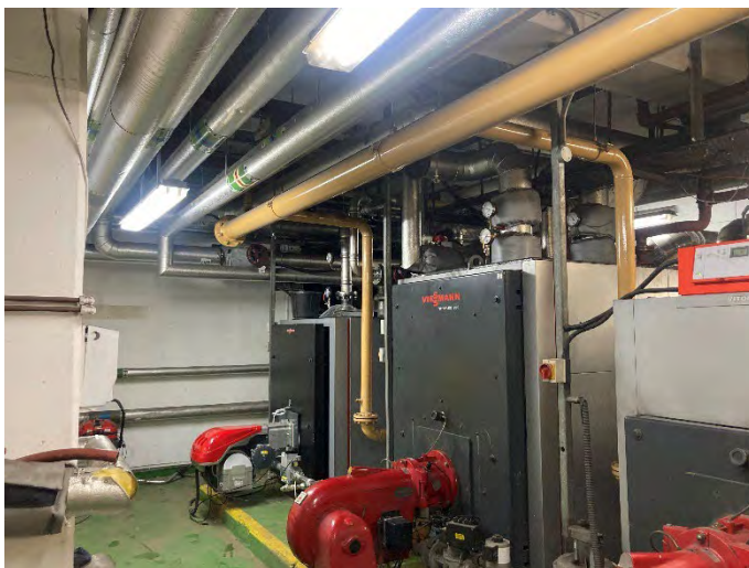
Photograph 7: MMU Library basement interior
