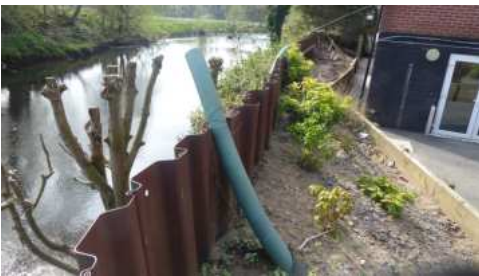
Figure 1.2: Sheet Piled Wall
