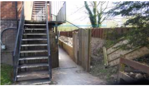
Figure 1.1: Sheet Piled Wall
