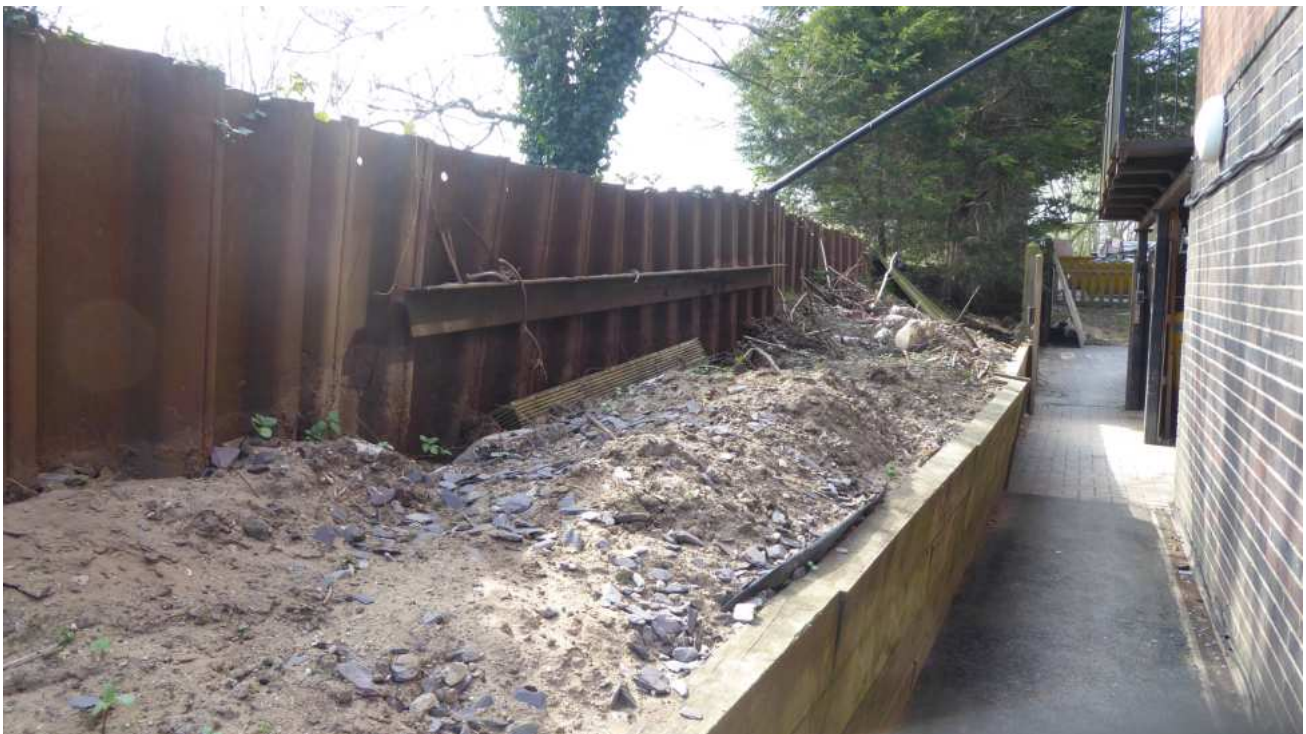
Figure 1.3: Sheet Piled Wall
