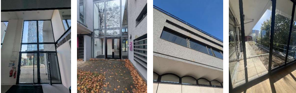
Existing Curtain Wall and Windows
