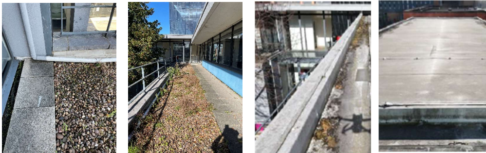
Existing Roof Finishes Low level terrace (left) and Upper Roofs (right)
