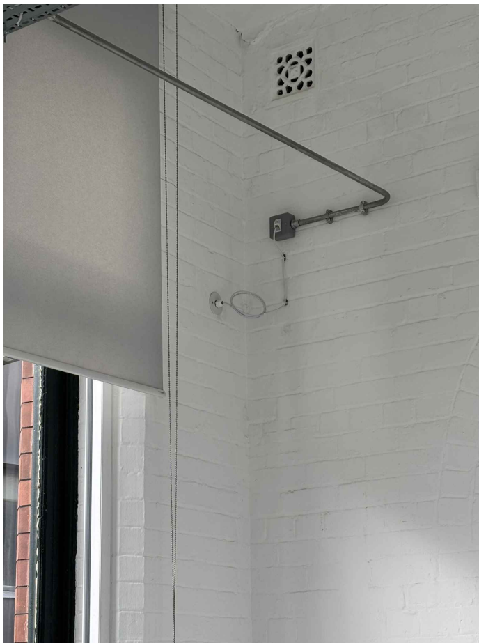
IMAGE 3 - EXTERNAL INSTALLATION METHOD OF EXTERNAL SERVICES
