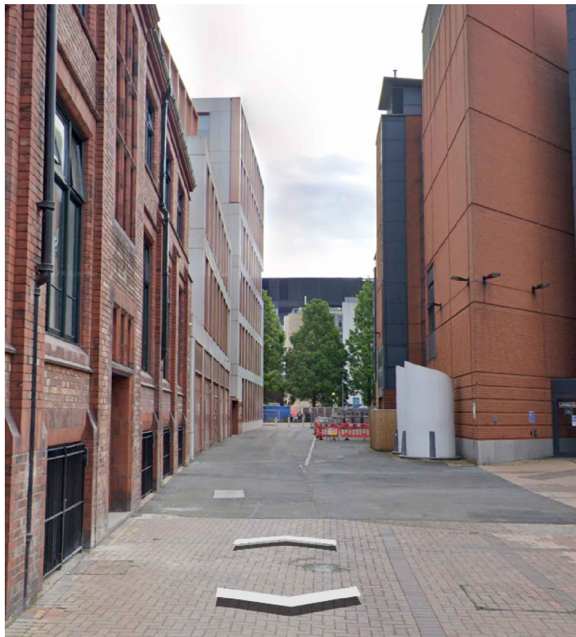
IMAGE 2 - EXTERNAL ELEVATION EXISTING FLOODLIGHTS ON BUILDING OPPOSITE
