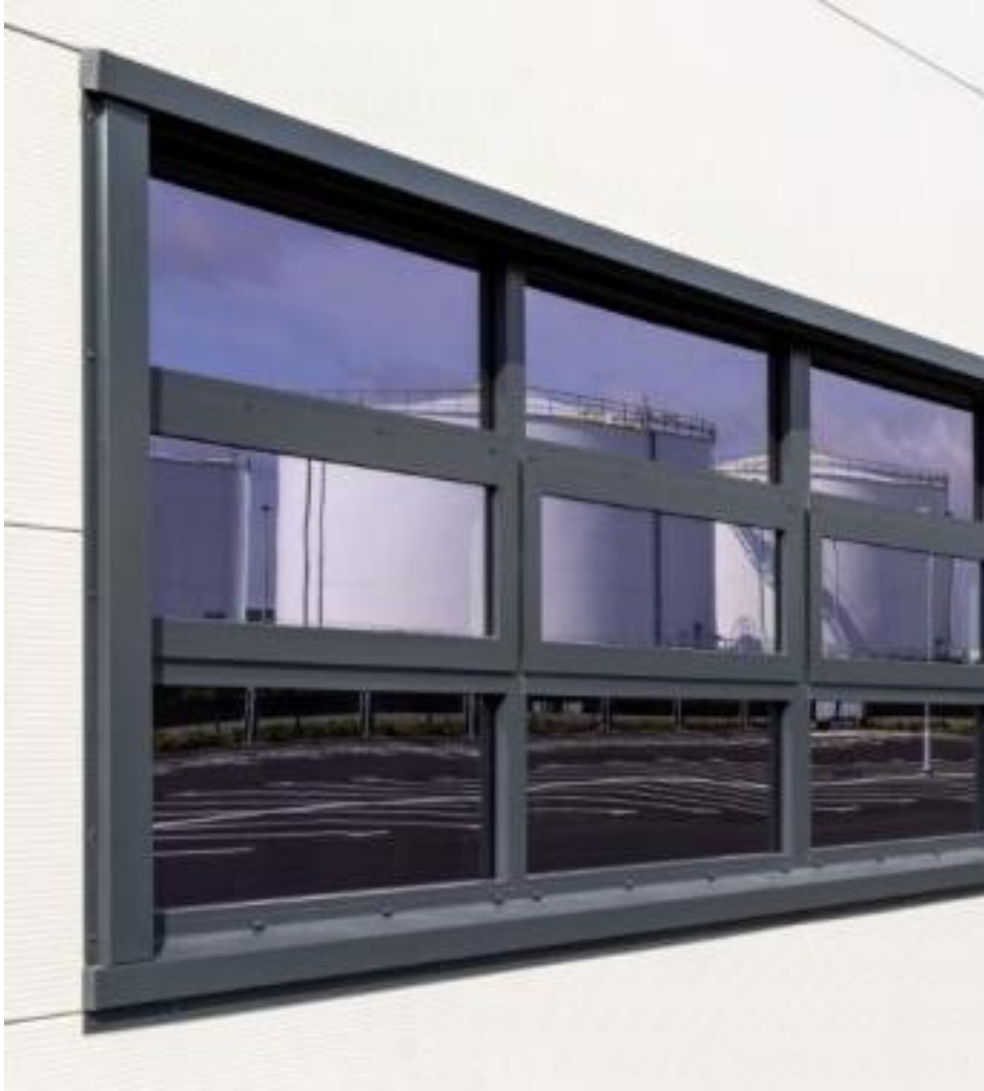
Aluminium feature band flashing (IV): Colour: Anthracite (RAL 7016)
