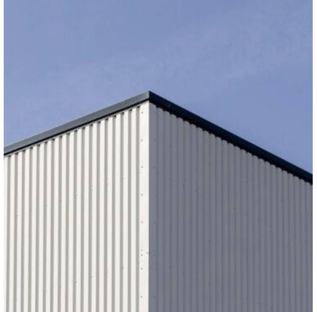
Aluminium parapet flashing (IX) Colour: Anthracite (RAL 7016)
