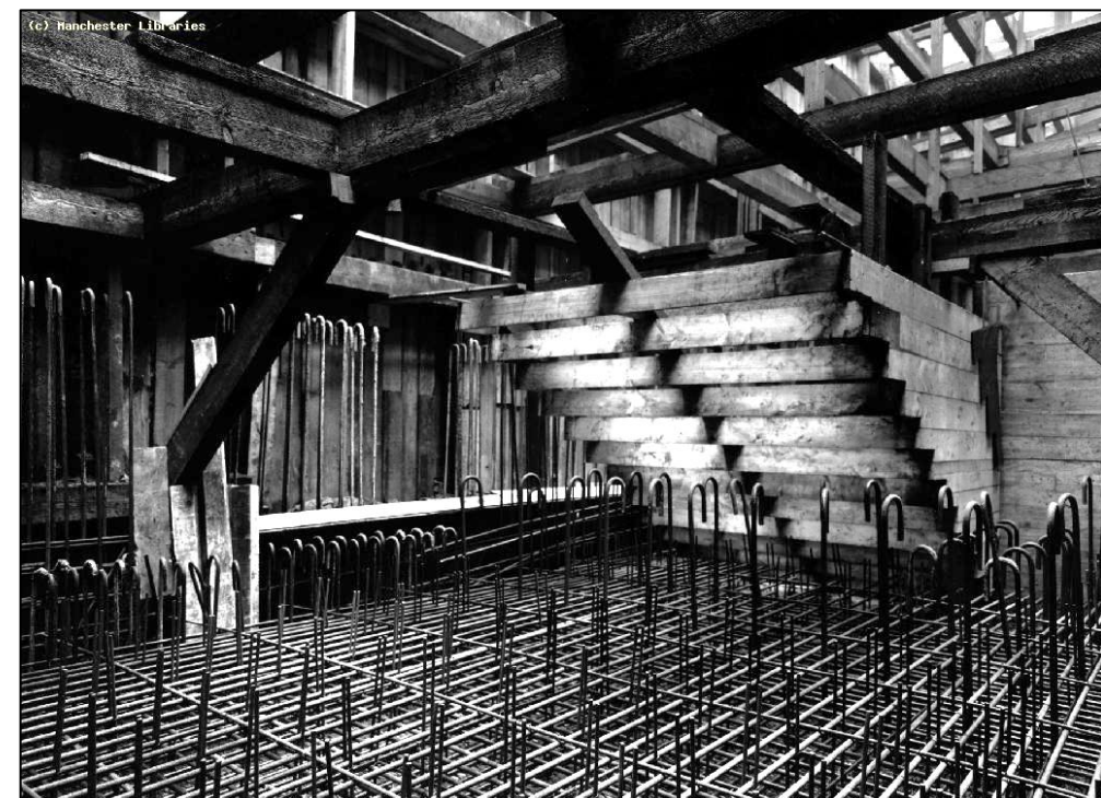
Figure 7 : The Bunker under construction, 1940. Image © Manchester Libraries
