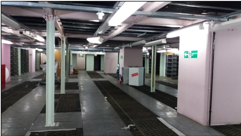
Figure 10 : Basement under the Tower showing RC columns and also 'temporary' steel structure
