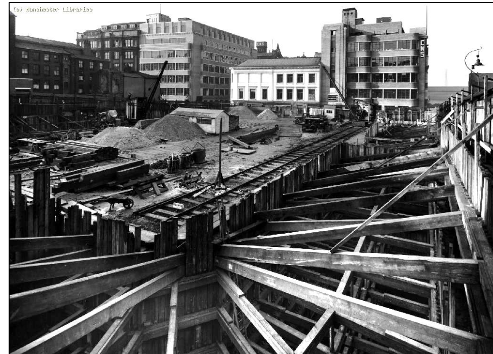
Figure 6 : The Bunker under construction, 1940 (looking towards Dantzic Street). Image © Manchester Libraries
