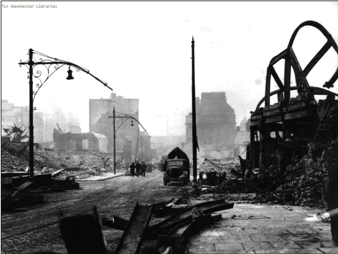
Figure 4 : Destroyed buildings on Miller Street following bombing raids in December 1940. Image © Manchester Libraries
