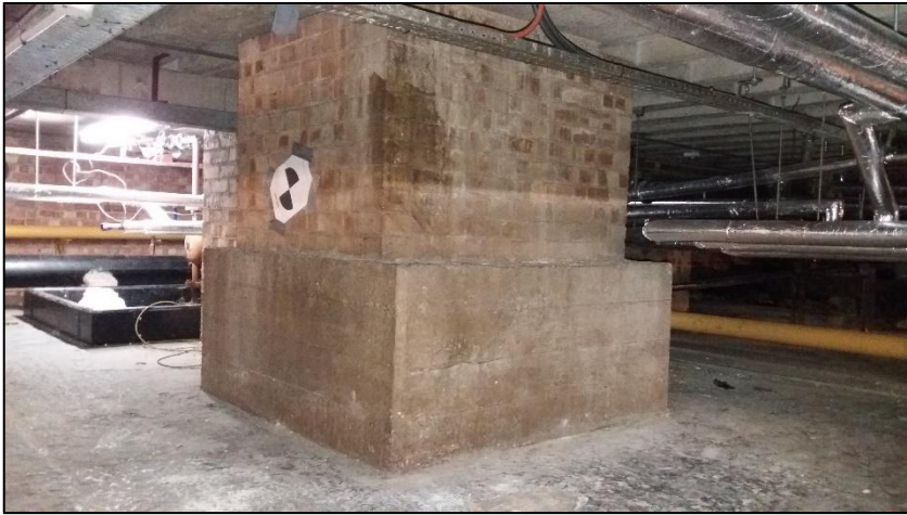
Figure 9 : Podium column founded on the bunker roof
