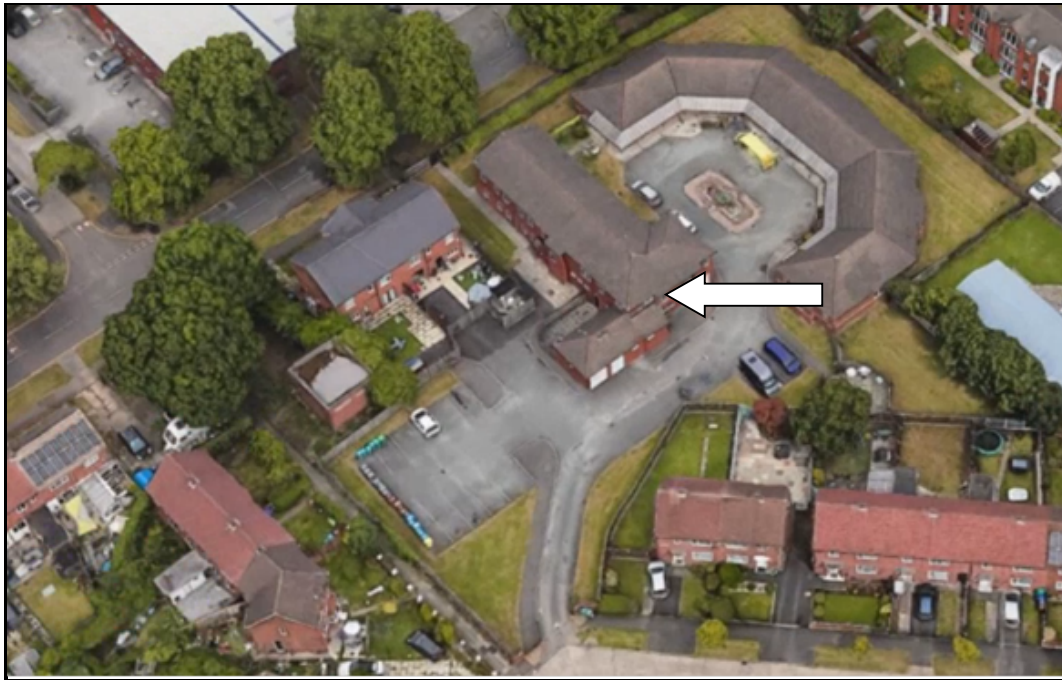
Aerial view of application site. Relevant building indicated by arrow
