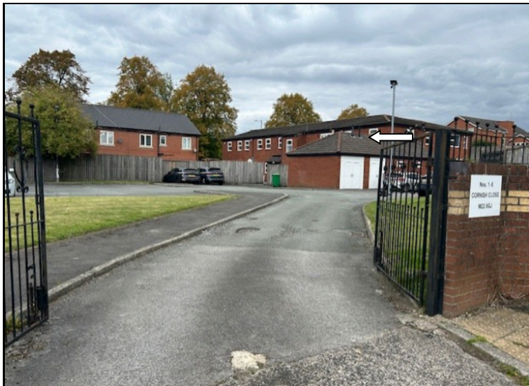
View of application site
