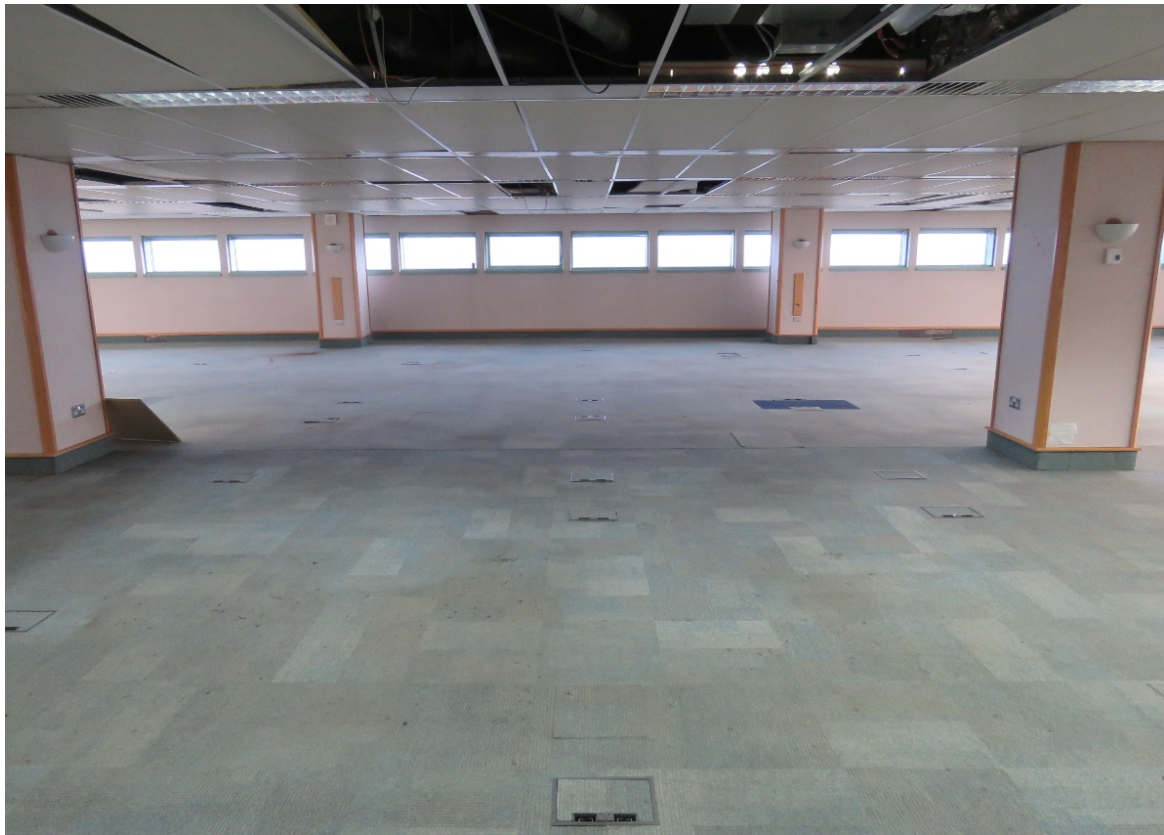
25-01 Looking north across the space, showing the inserted ceilings, floors and column cladding.
