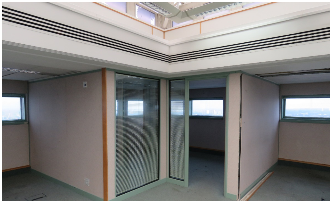
25-11 Detail of the inserted south-west partitioned offices.
