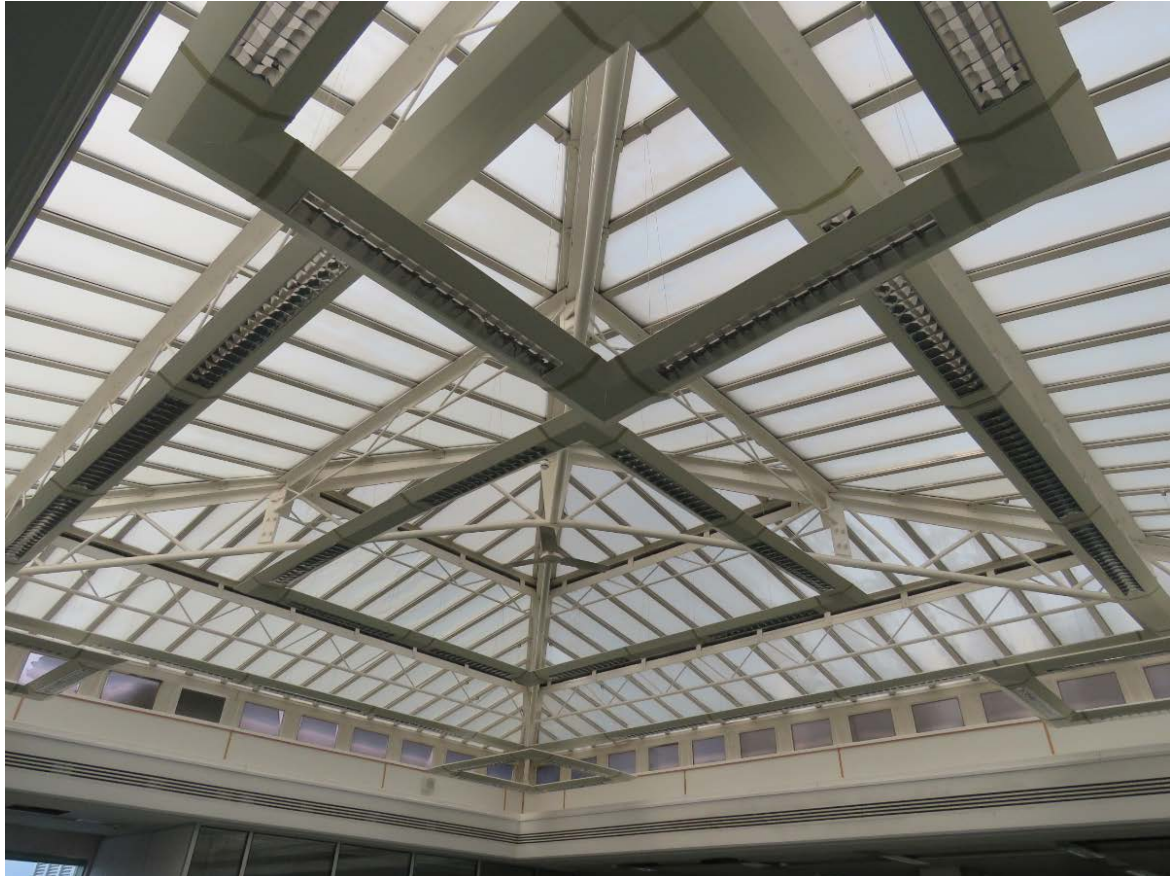
25-04 The underside of the east-end pyramid roof-light, showing the applied film and new lighting which changes the lighting and removed the vertical views.
