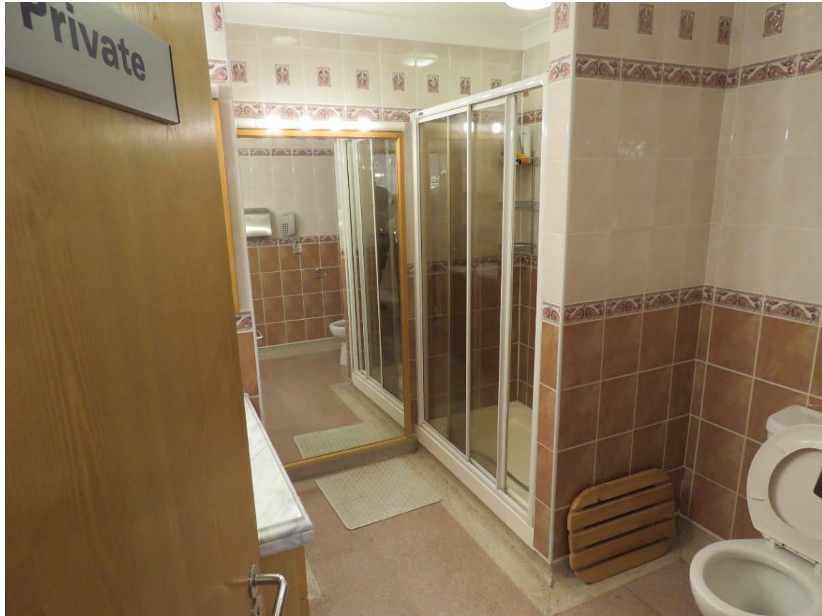
25-08 Interior details of the north-east executive bathroom. Non-original fixtures and fittings.
