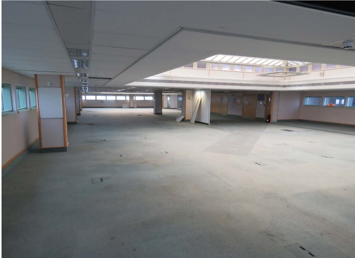
25-02 Looking south-east towards the entrance, showing the underside of the altered roof-light.
