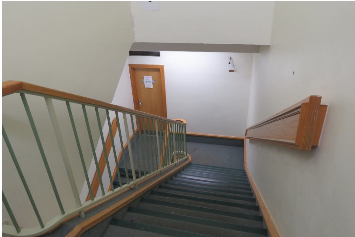
25-06 North-east stairs down to the executive bathroom and 24 th floor.
