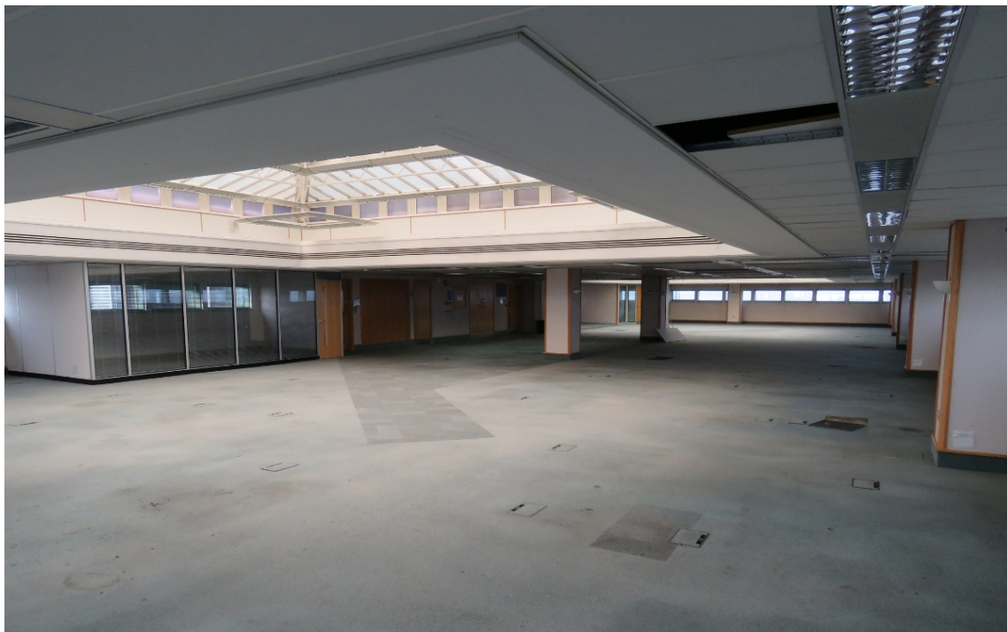
25-03 Looking south-west towards the entrance, showing the underside of the altered roof-light and the inserted office partitions.
