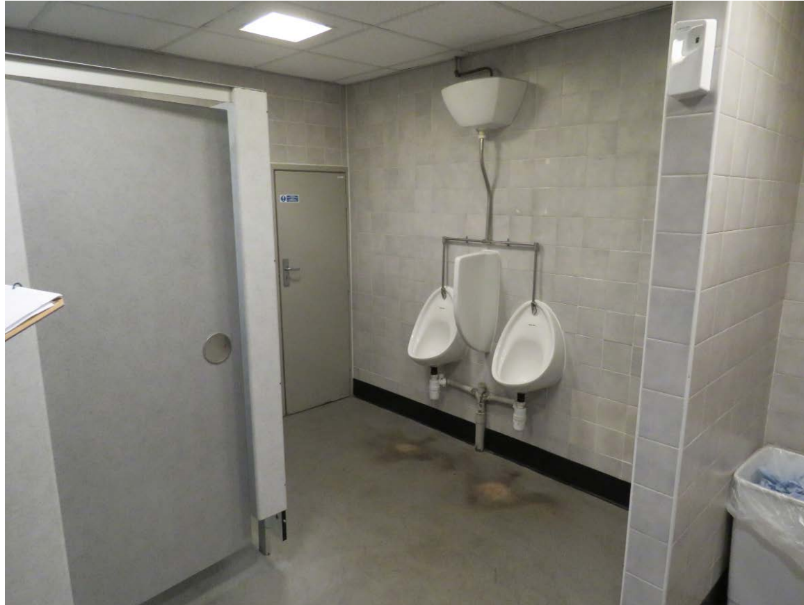
25-10 Interior of the north-west toilets.
