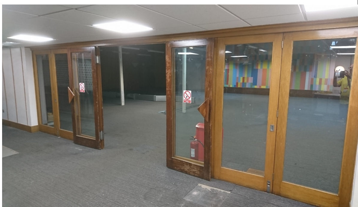
05-14 View of original glazed doors between the bar and recreation space.
