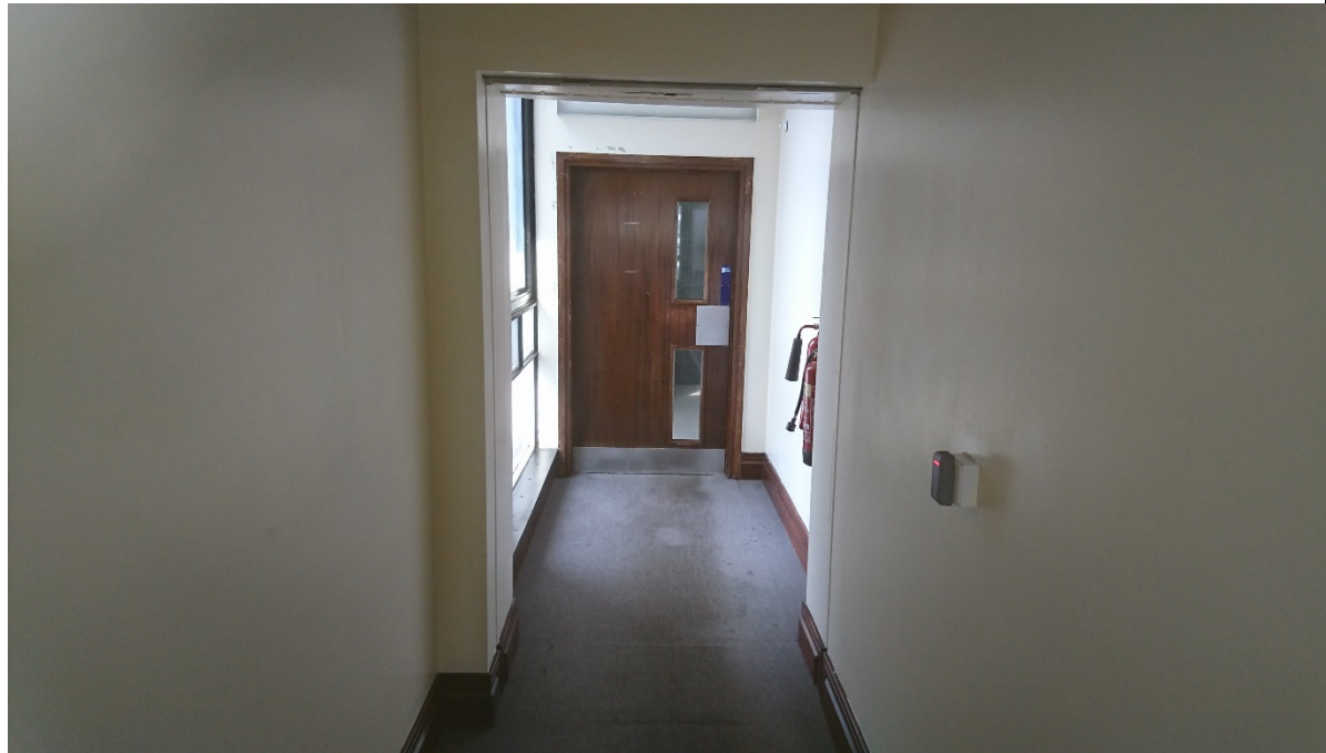
05-06 View of corridor leading to the east stairwell.
