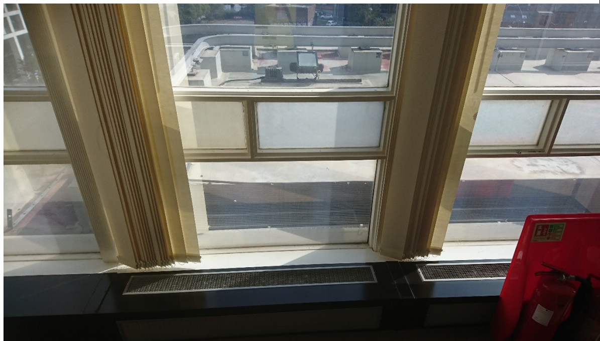
05-05 View of windows with original timber bead to glazing and perimeter weathermaster.
