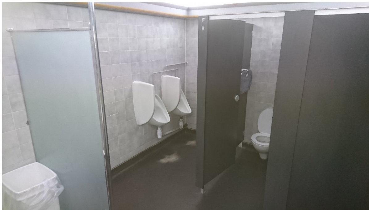
05-09 View of gents WC with original glass screen, non-original cubicles and vinyl over original floor finish.
