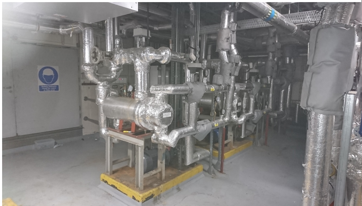
05-23 View of the eastern plant room looking south.
