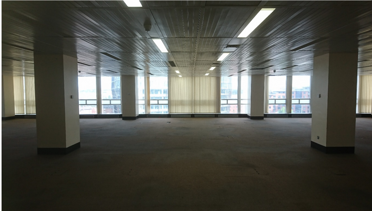
05-02 View on entering the office area looking north towards the Miller Street Elevation.
