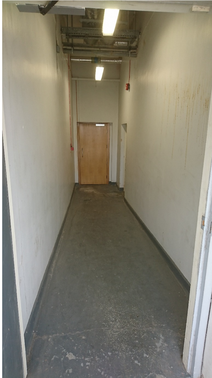
05-28 View east back along the corridor to the roof of the podium.
