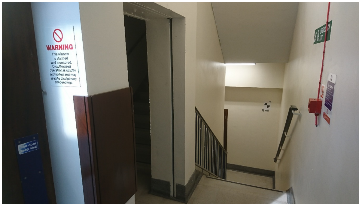
05-07 View of east stairwell with fire compartmentation.
