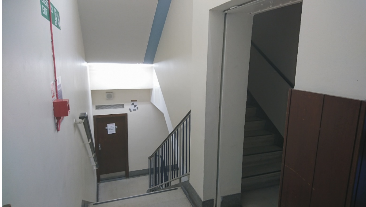
05-08 View of west stairwell with fire compartmentation.
