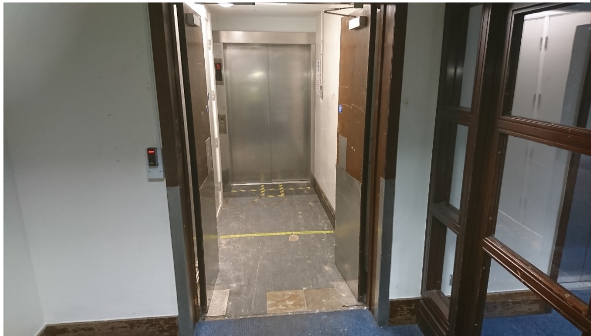
05-11 View west into the service lift.
