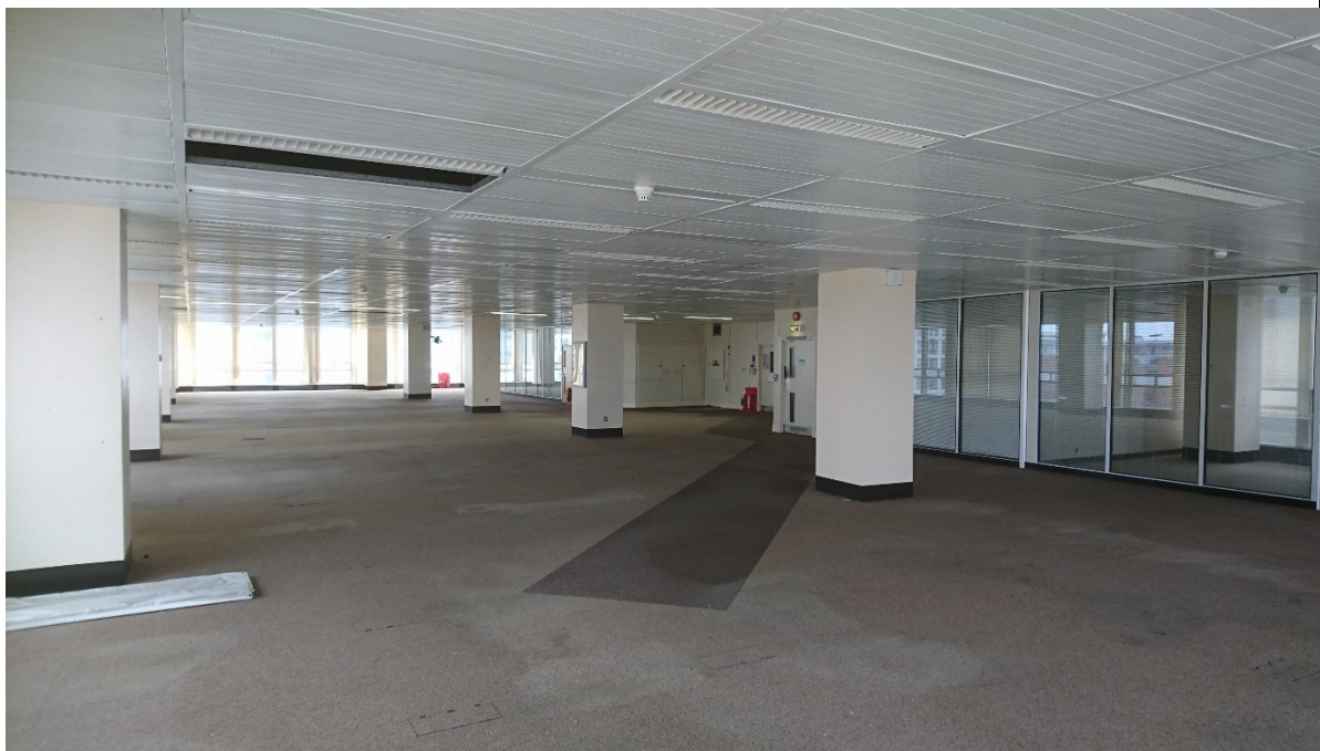
05-03 View looking back south across the office accommodation with glazed partitioning to separate meeting / office space.
