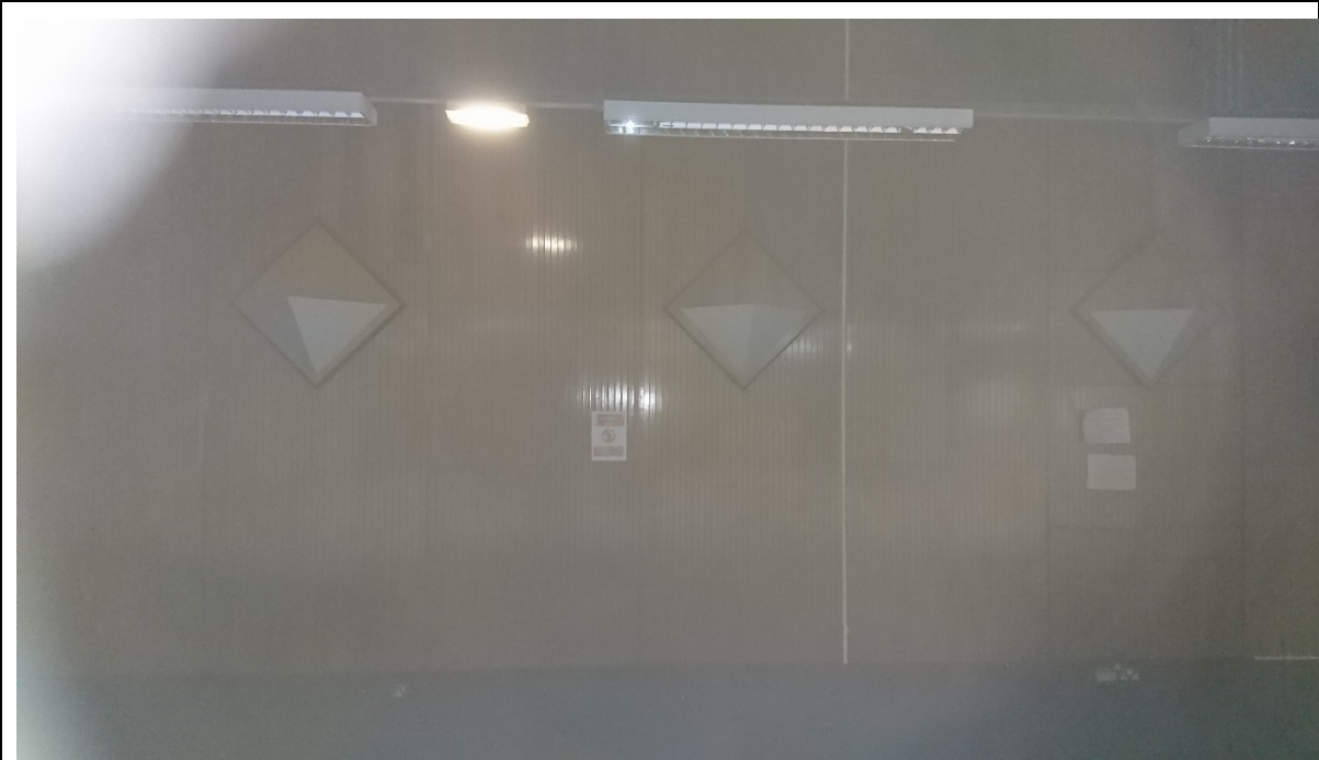
05-20 View of the west wall of the recreation space showing the non-original acoustic panels and wall lighting.
