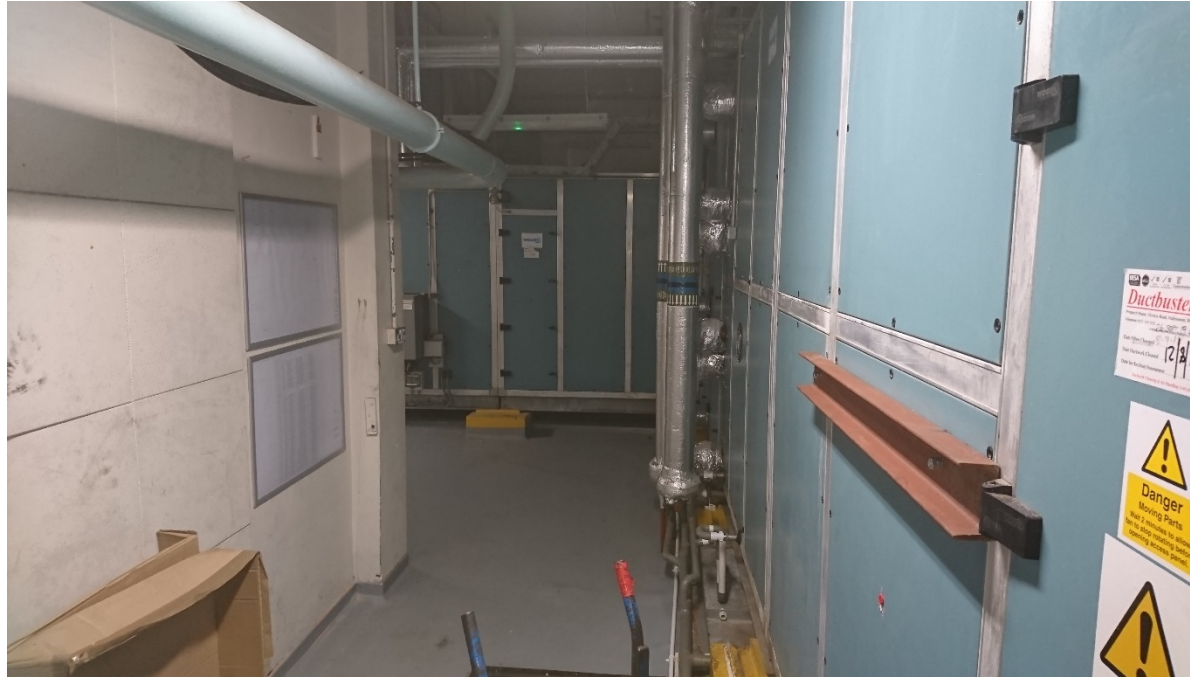
05-24 View of the eastern plant room looking north.
