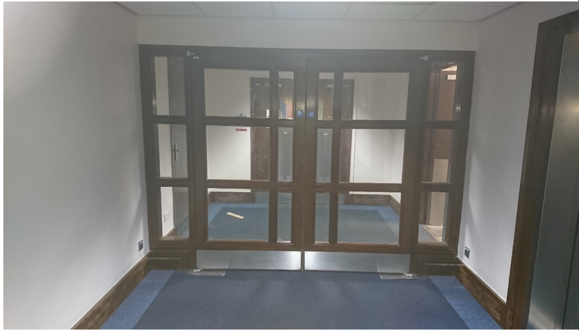
05-10 View south in lift lobby with original doors.
