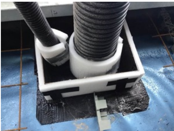
Sealed pipe penetrations
