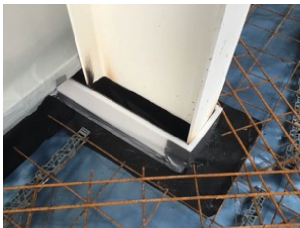
Sealed stanchion detailing
