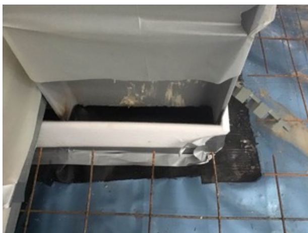
Sealed stanchion detailing
