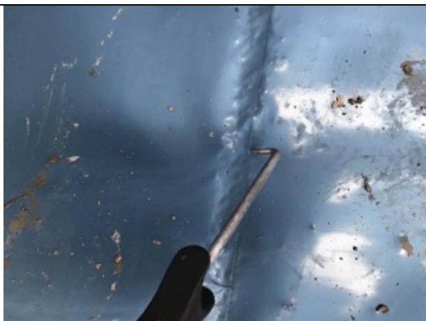
Hand weld probe testing
