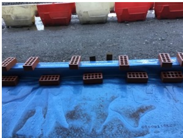
Unit 3 membrane extended over the perimeter edge
