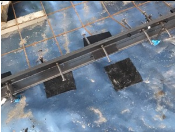
Sealed patch repairs
