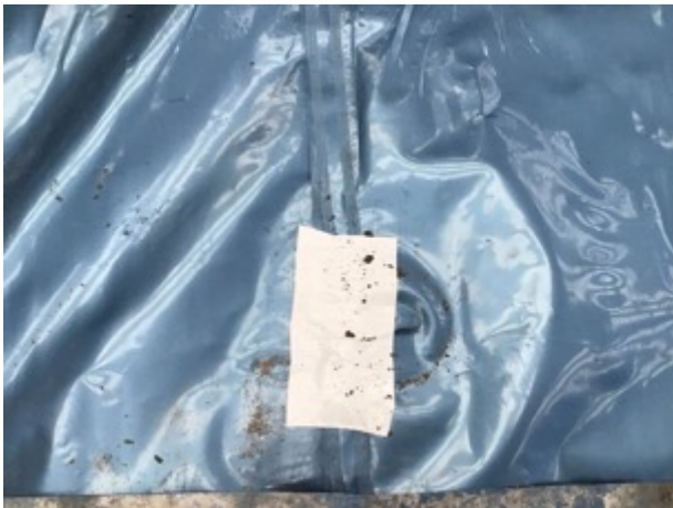
Sealed patch repair
