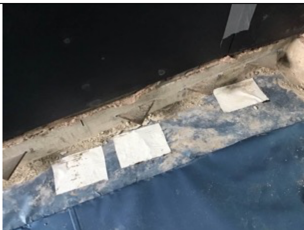
Unit 2 patch repairs
