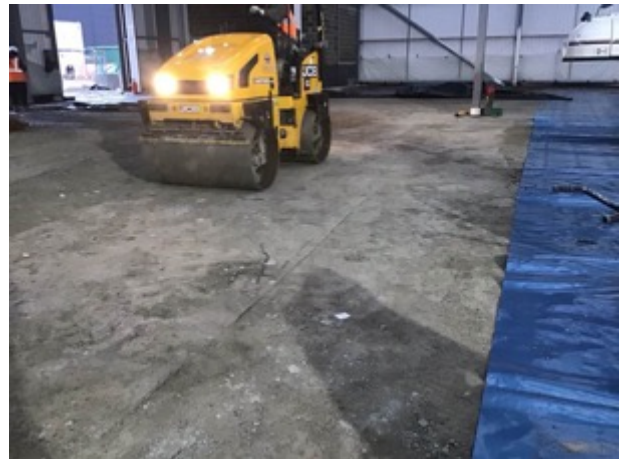
Sub grade prep
