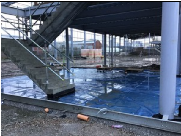
Unit 2 core area line out installation
