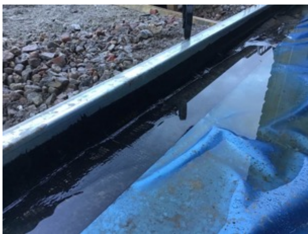
Sealed perimeter retro fit detailing
