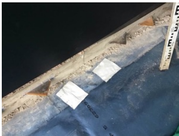
Unit 3 patch repairs
