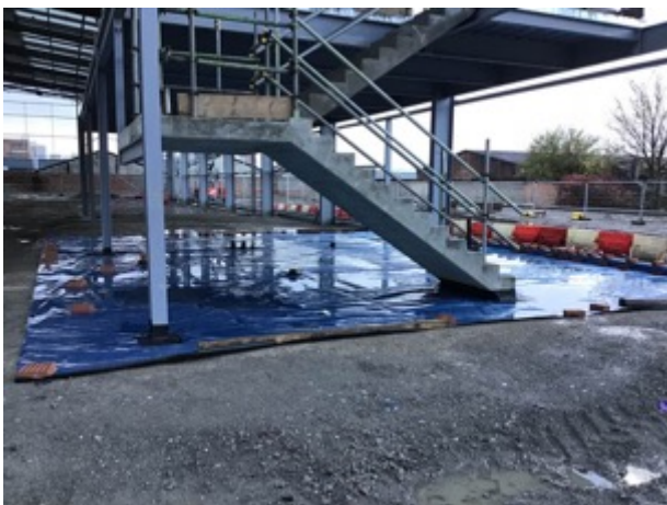
Unit 3 core area line out installation
