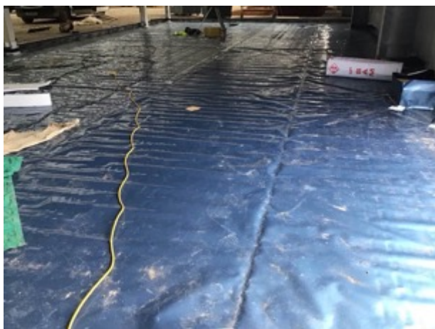
Unit 3 undercroft overview
