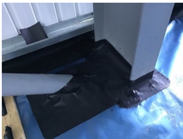
Sealed stanchion detailing
