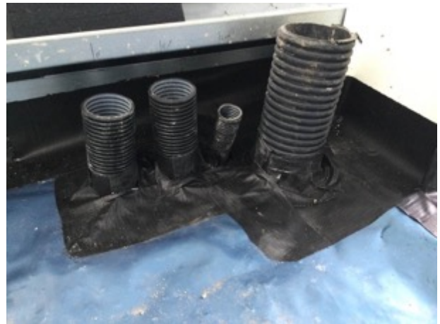
Pipe penetration details sealed using SAGM.
