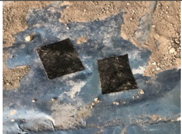
Sealed SAGM patch repairs
