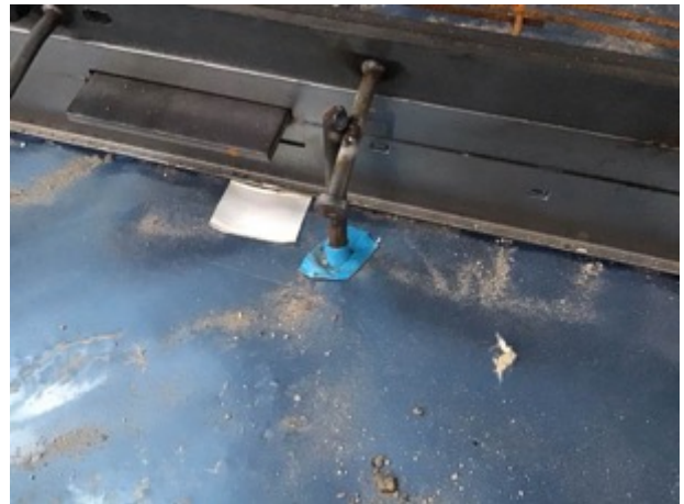
Butyl tape on armoured joint pin
