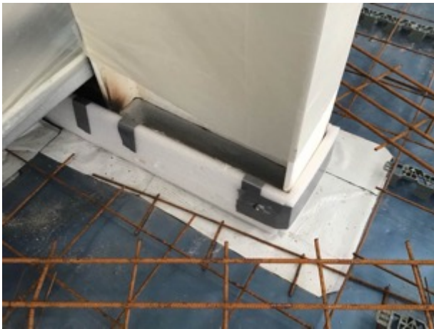
Sealed stanchion detailing
