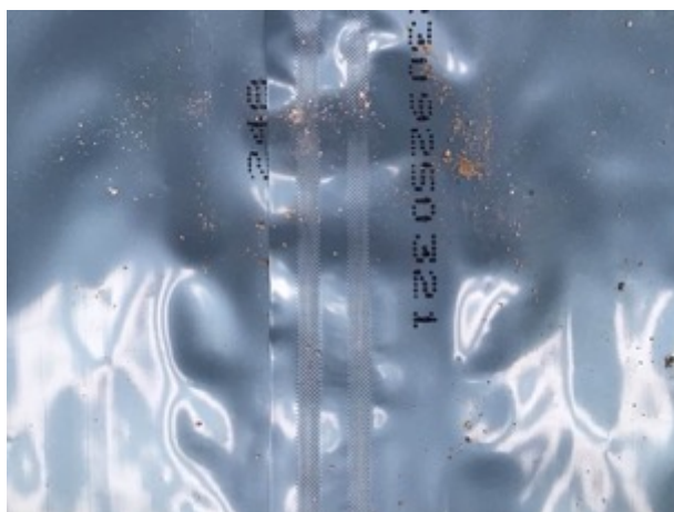
Auto weld membrane joint
