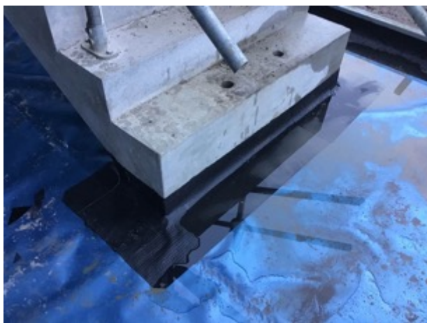
Sealed retro fit detailing to stairs
