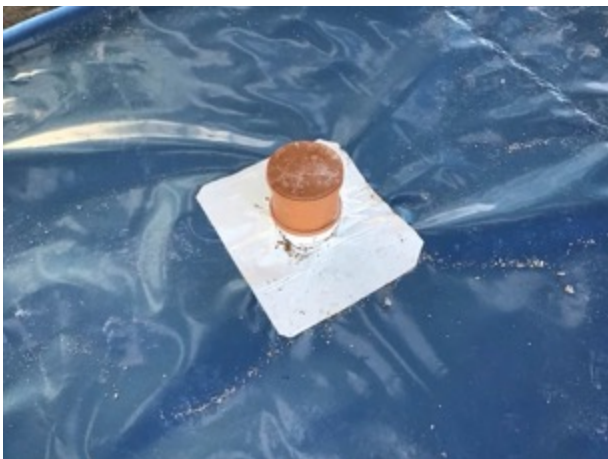
Core 7 sealed pipe penetration
