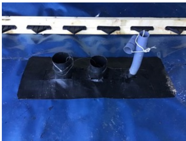
Sealed pipe penetrations
