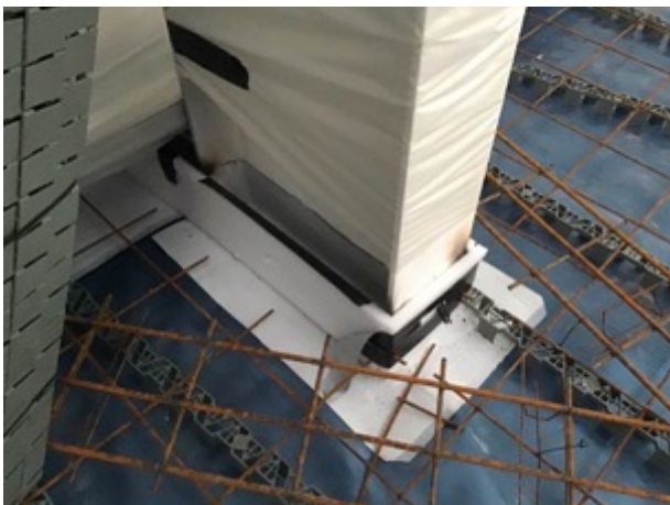
Sealed stanchion detailing
