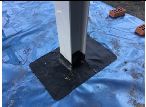
Unit 3 sealed stanchion detailing
