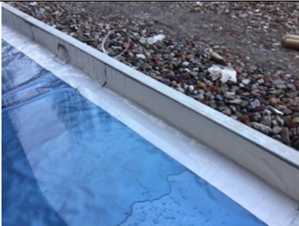
Core 8 sealed perimeter retro fit detailing
