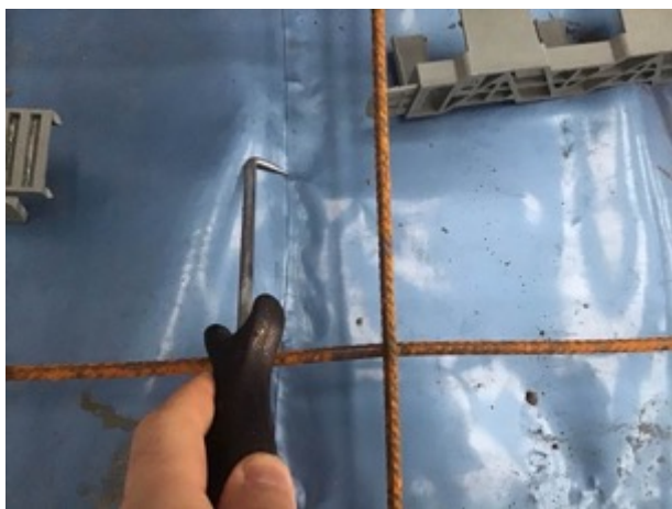
Probe test on hand weld
