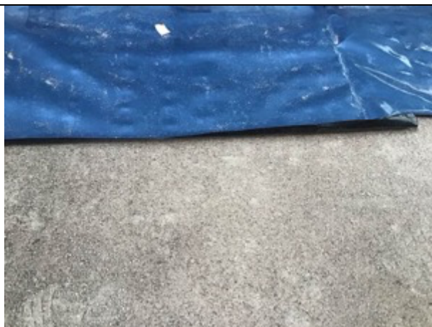
Rolled sub grade
