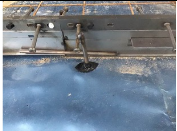
Armoured pin sealed with butyl tape
