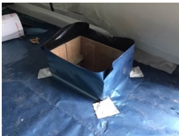
Unit 3 boxed out area
