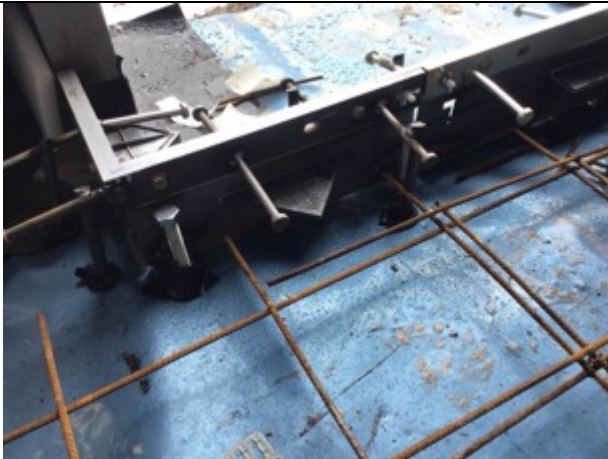
Armoured joint pins sealed using butyl tape
