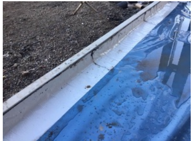
Core 4 sealed perimeter retro fit detailing
