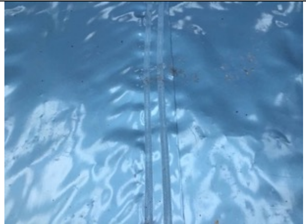
Auto weld membrane joint
