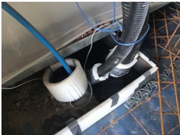
Sealed pipe penetrations
