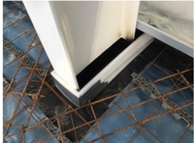
Sealed stanchion detailing
