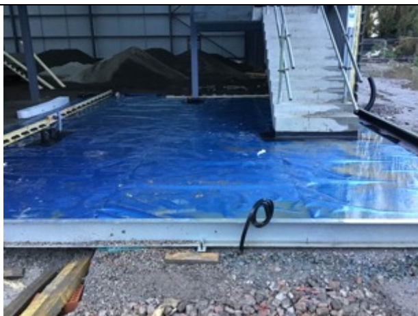
Unit 9 core area line out installation
