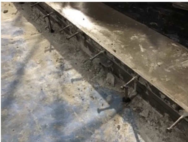
Pins sealed with butyl tape
