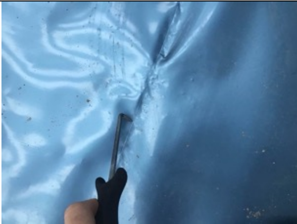
Probe test to hand weld
