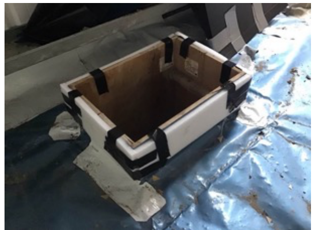
Unit 2 boxed out area
