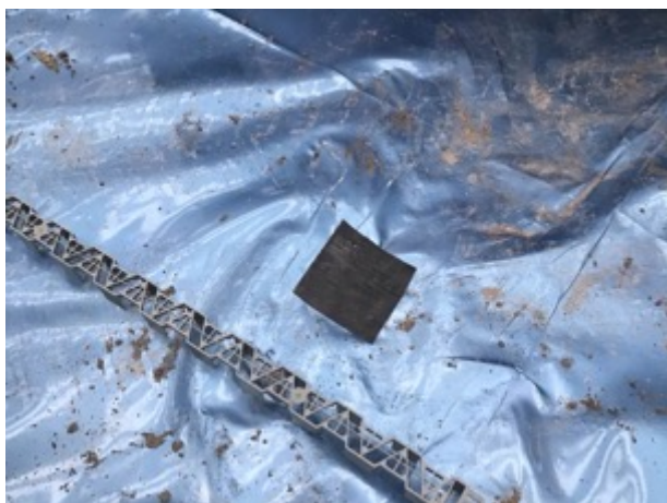
Sealed patch repair
