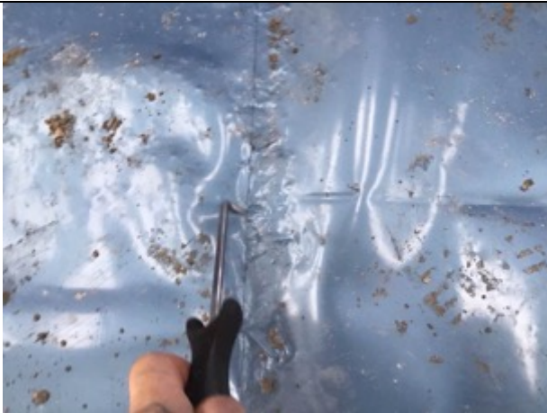
Hand weld probe testing
