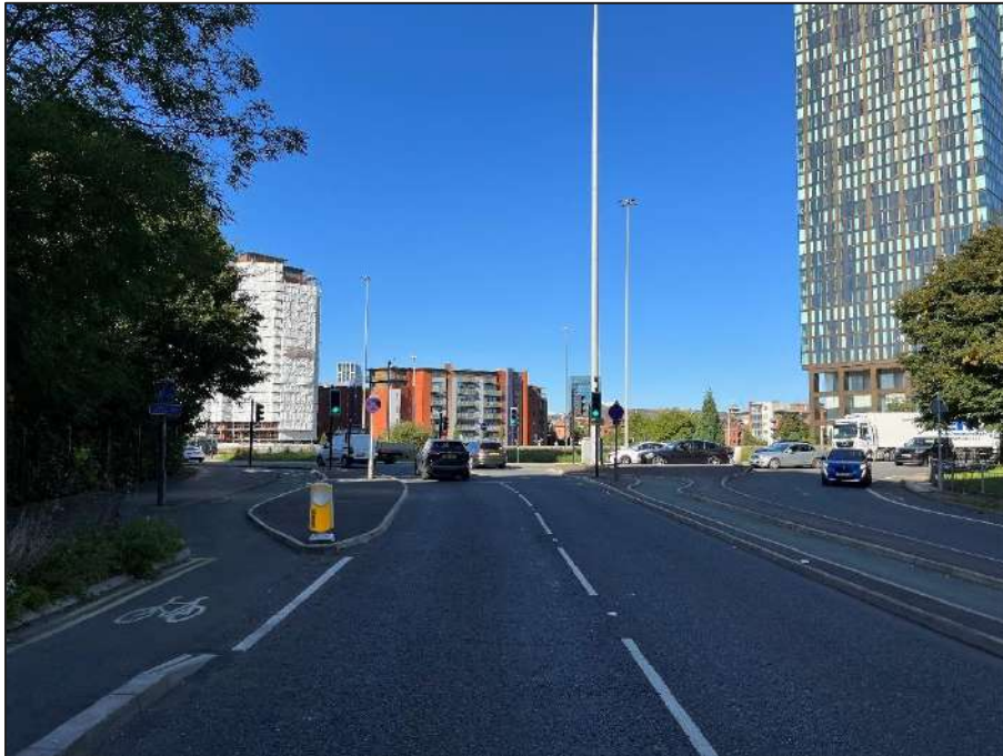
Figure 2.1 – A5067 Chorlton Road Approach to Deansgate Interchange
