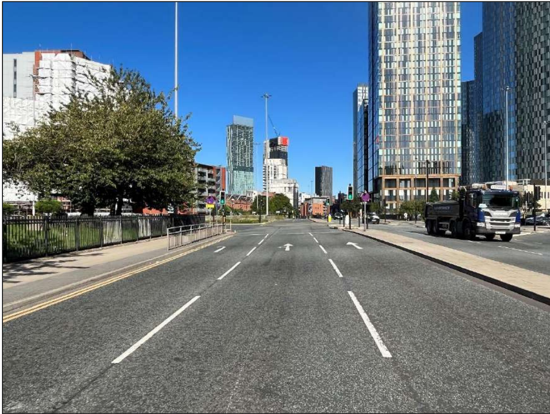
Figure 2.3 – A56 Chester Road (W) Approach to Deansgate Interchange
