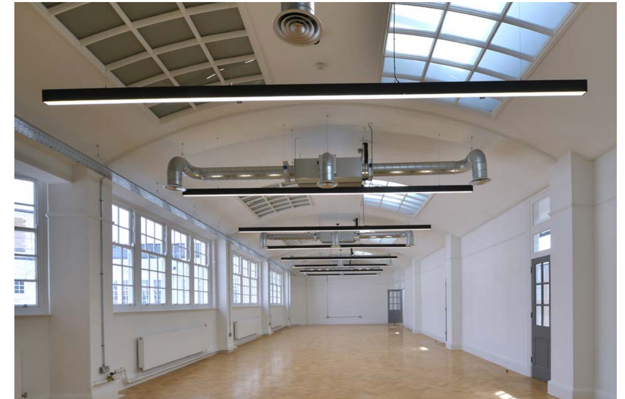
Existing arched ceiling on Level 13
