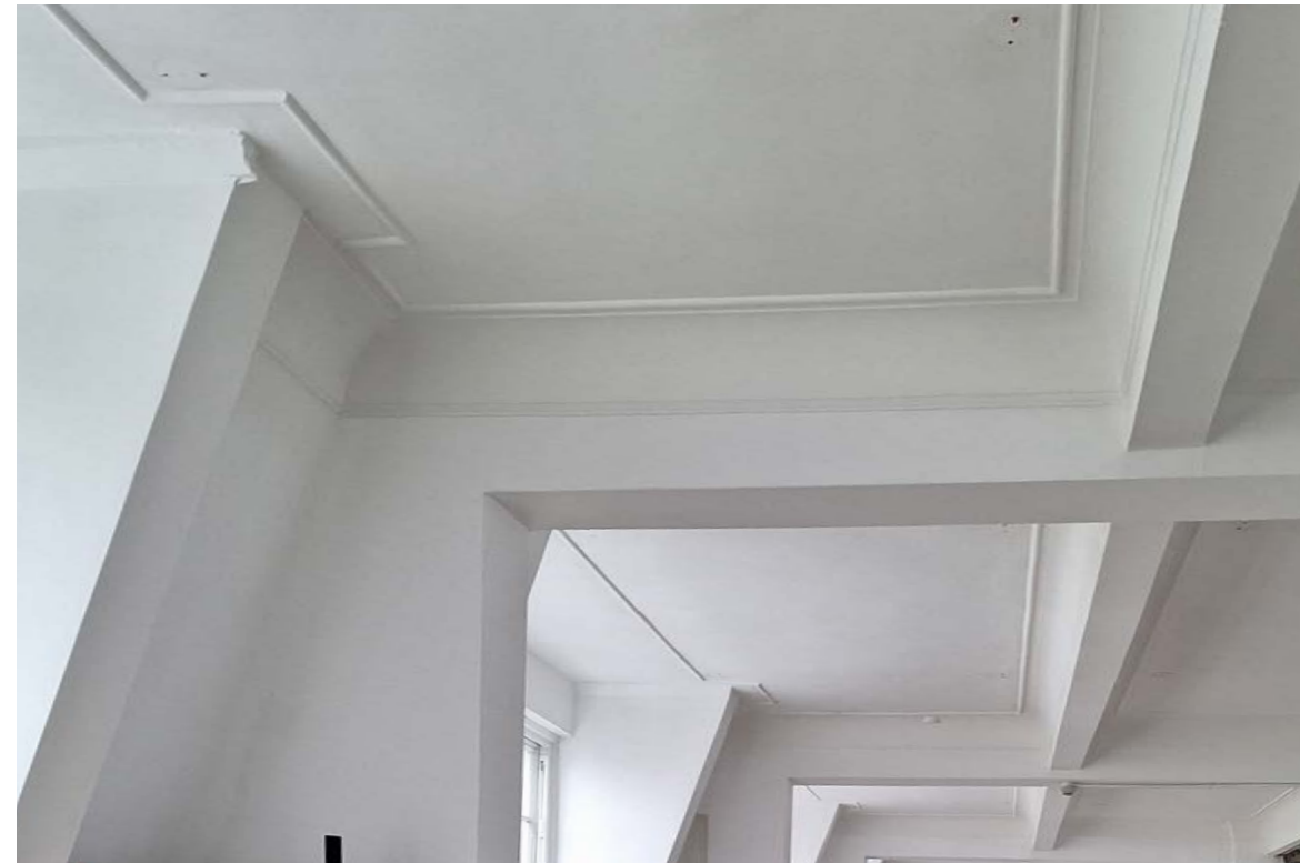
Existing coffered ceiling on Level 11
