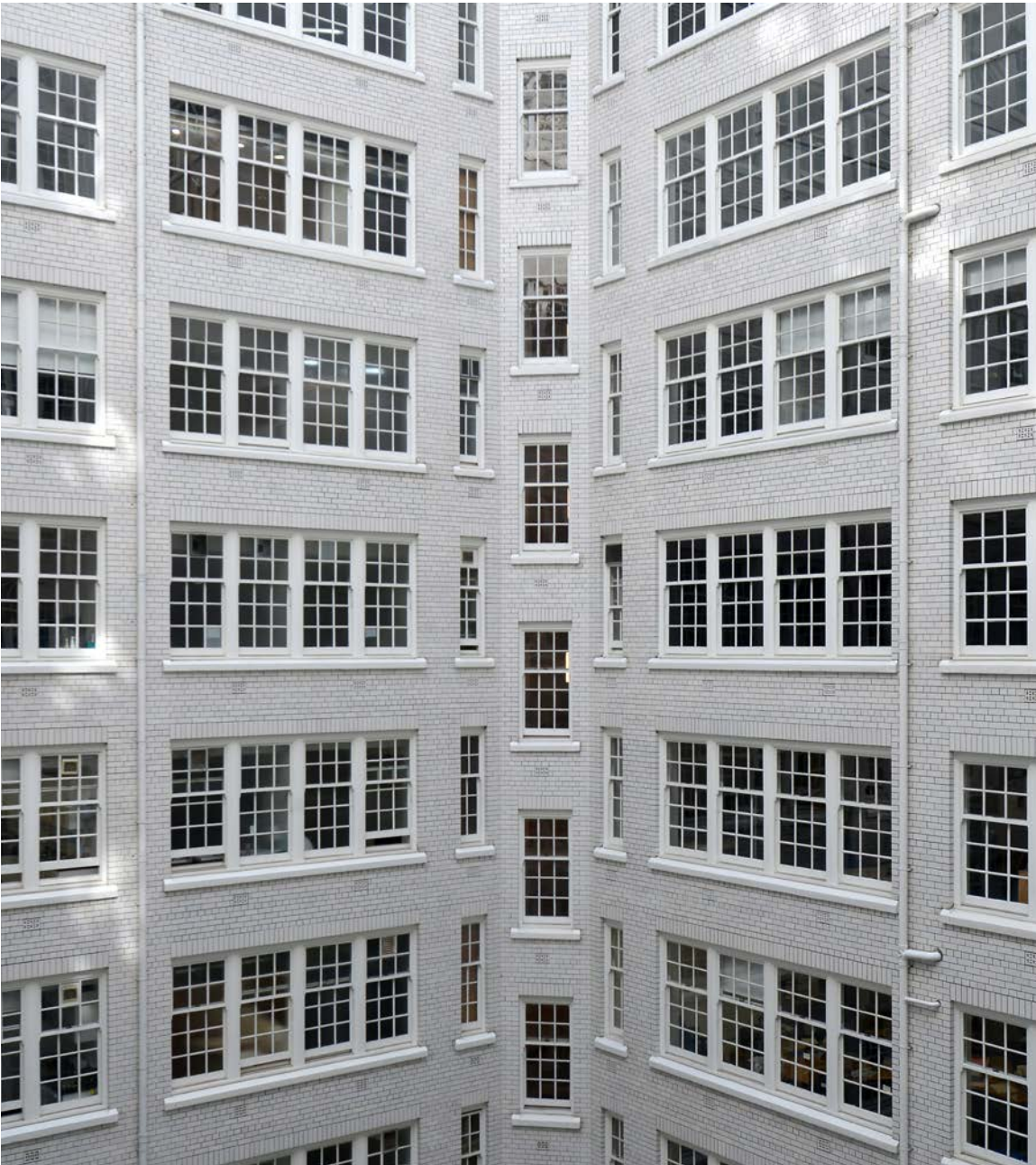
03 View of the internal atrium windows
