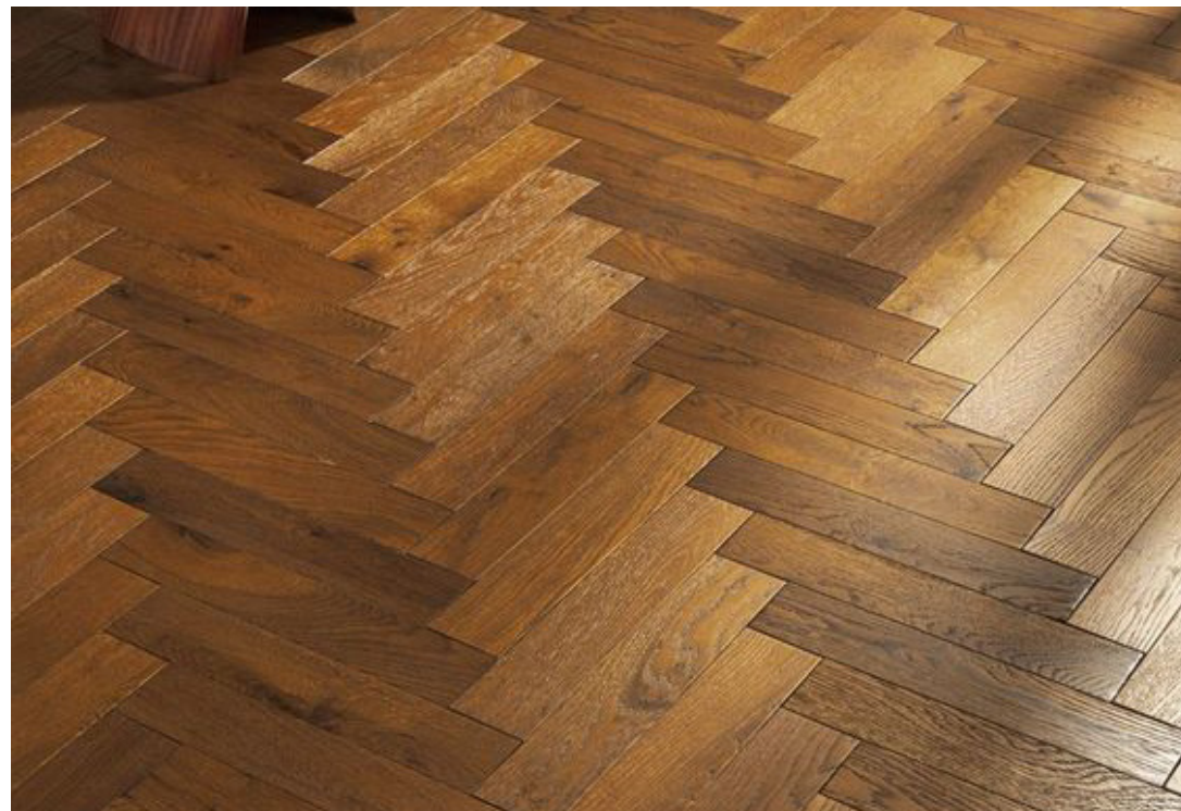
A. EXISTING PARQUET FLOORING
