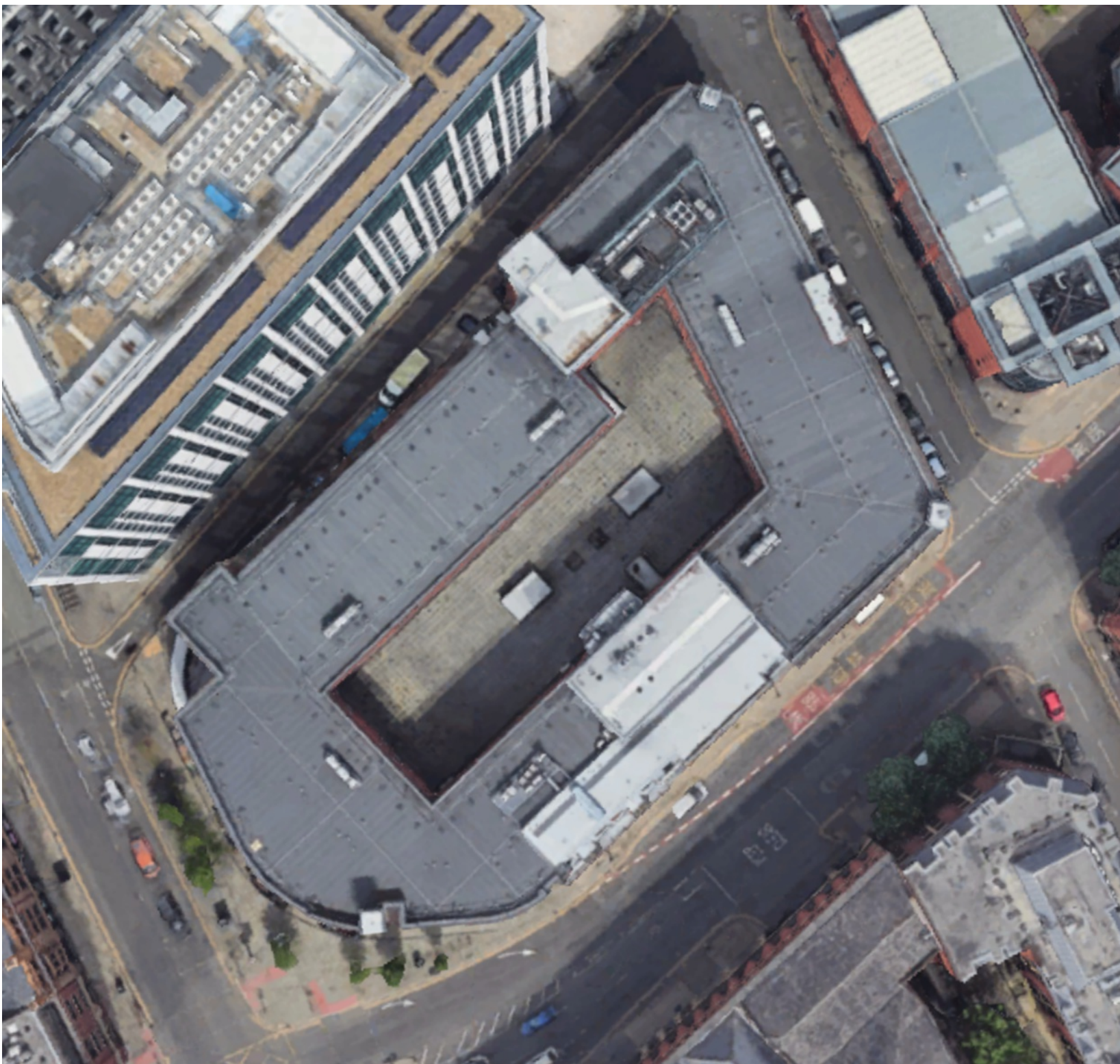
EXISTING ROOF (AERIAL IMAGE) NOT TO SCALE
