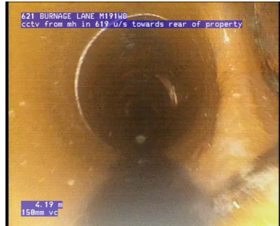
Photo: 6_6_53_A.jpg, 00:00:14 4.19m, Junction, at 3 o'clock, diameter 150mm
