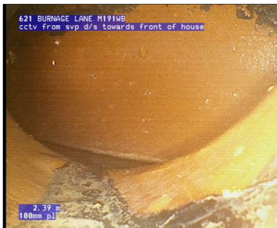
Photo: 1_1_9_A.jpg, 00:00:36 2.39m, General remark Remarks: Joining Carrier Line
