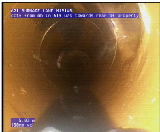
Photo: 6_6_54_A.jpg, 00:00:15 5.03m, Junction, at 2 o'clock, diameter 100mm
