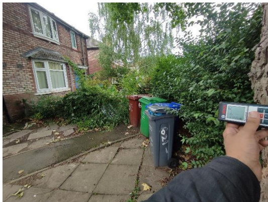
Photo 7 – The distance between the tree and neighbouring property which had previously been damaged and subsequently repaired was measured as 7.85m. The zone of influence of this tree is 19.5m.
