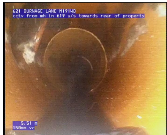
Photo: 6_6_55_A.jpg, 00:00:17 5.51m, Junction, at 10 o'clock, diameter 100mm
