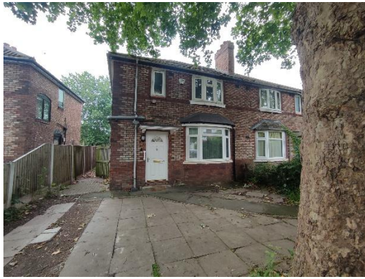
Photo 13 – View of the front elevation of the property
