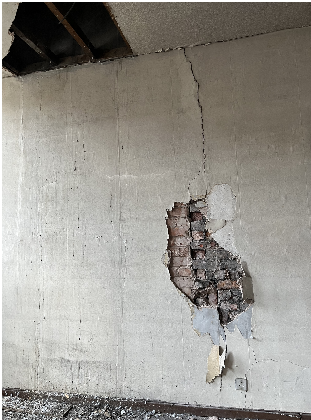
IMG_0427 (First Floor - Warwick St return wall)
