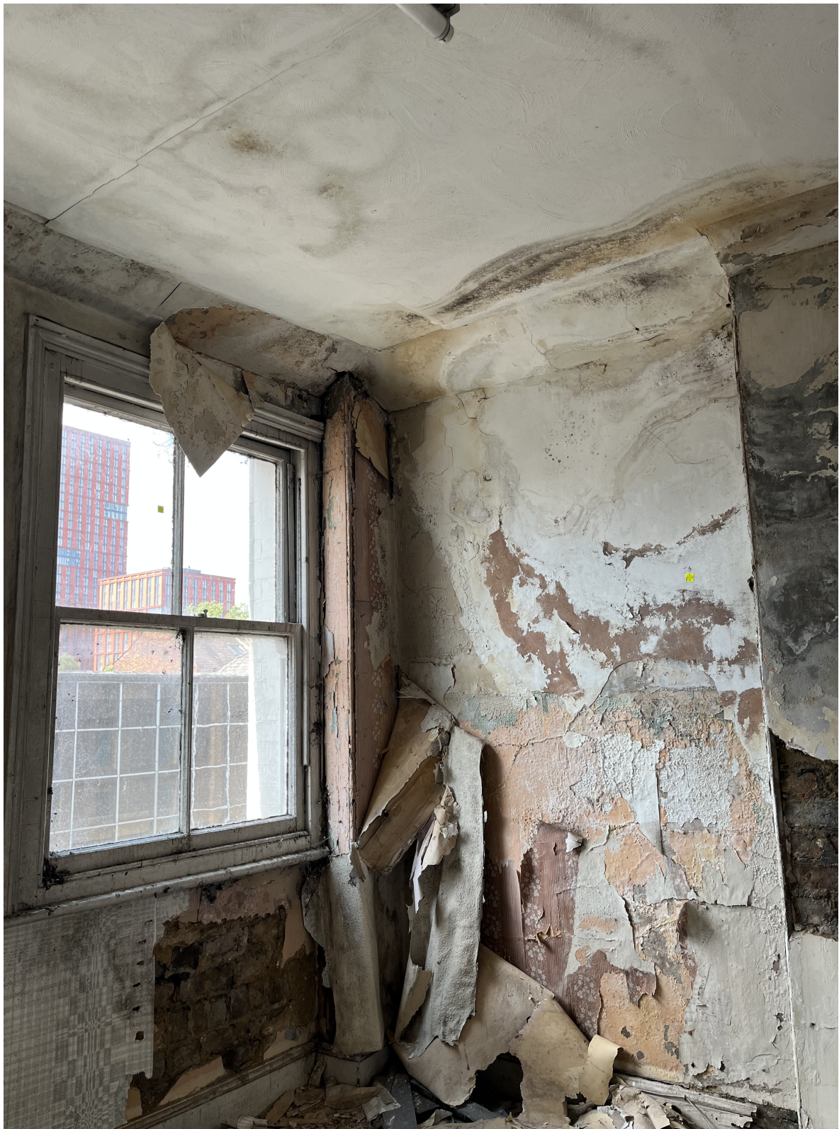
IMG_0461 (Second Floor - Warwick St return wall)
