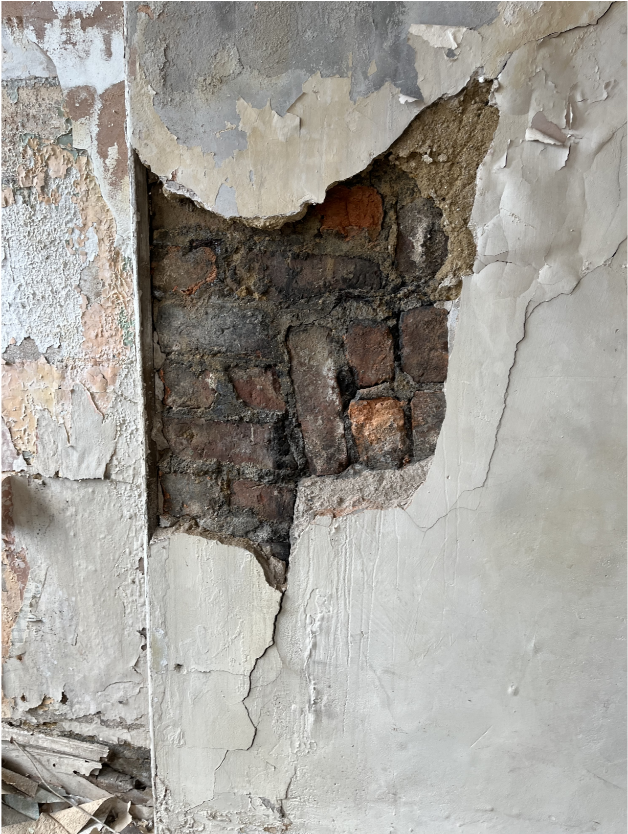
IMG_0463 (Second Floor - Warwick St return wall)
