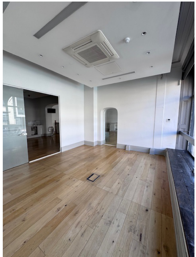
Image 7 First Floor Ceiling Raft.
