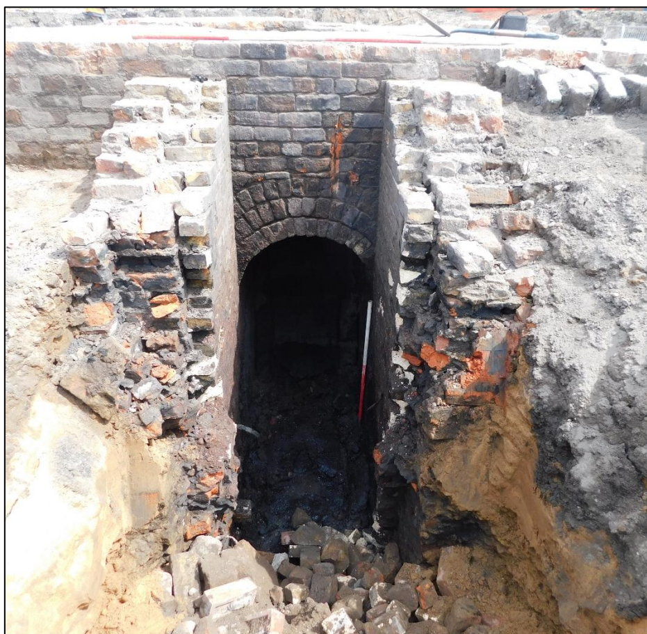
Plate 23: Flue 026 in the south-west of chimney 005, bounded by structure 008, showing the depth of the flue
