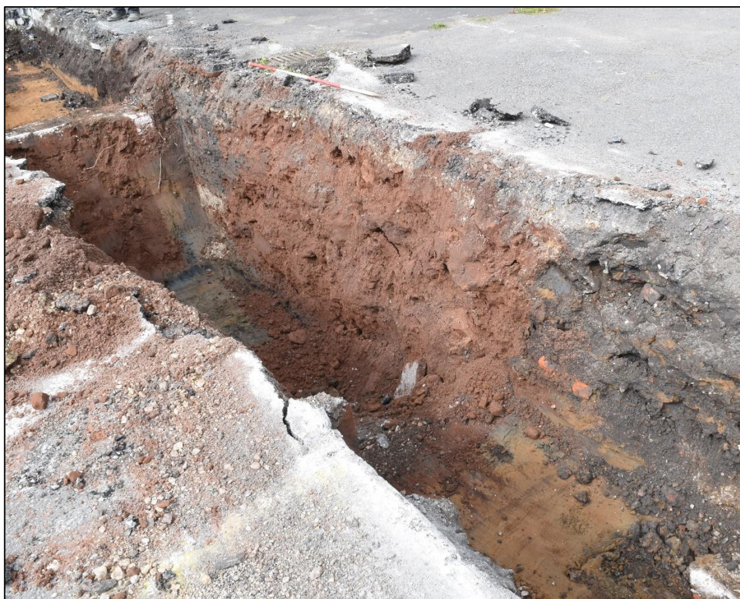
Plate 10: Modern cut [202] filled by (204), looking broadly north
