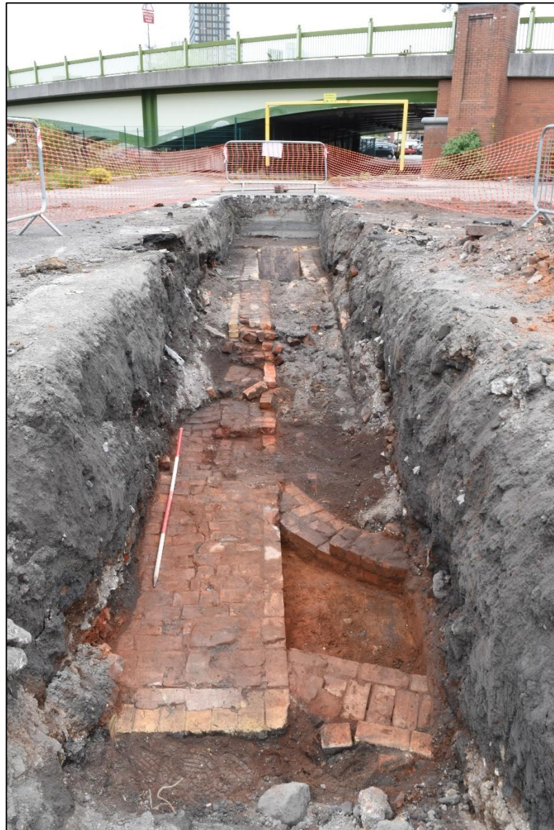
Plate 8: View of engine bed 109 and flue, looking north-east
