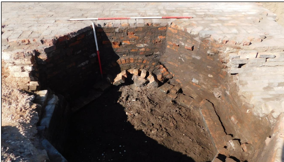
Plate 22: Arch in the north-east elevation of chimney 005, looking north-east
