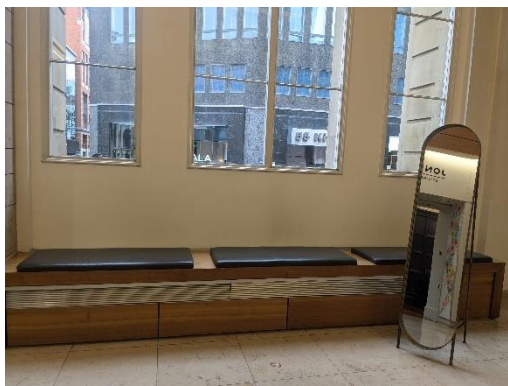
Figure 16: Non-historic joinery with integrated ventilation system in reception area.
