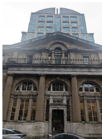
Figure 9: View of the 1990s tower extension above the historic building from King Street.
