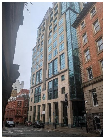
Figure 8: View of the 1990s tower extension to 82 King Street from Tib Lane.
