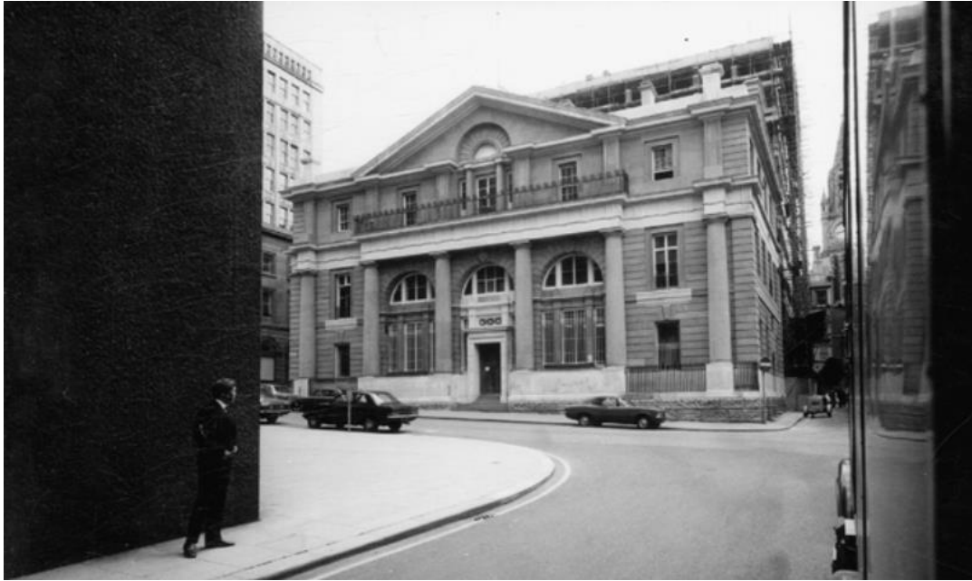
Figure 26: Former bank viewed from Cheapside, 1972. There was evidently a building constructed to the rear of the bank in this period, replaced by the 1995 tower extension. Source: Greater Manchester Lives.
