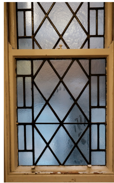
Figure 17 Upper Floor Lightwell Windows
