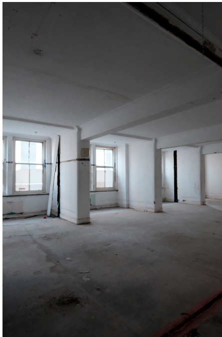
Figure 12 Upper Floor Space
