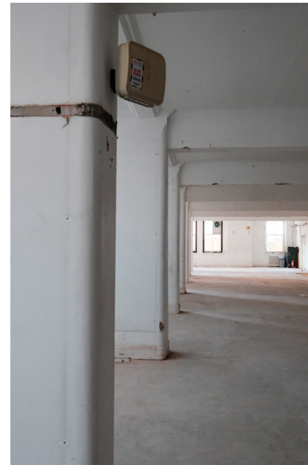
Figure 15 Upper Floor Space
