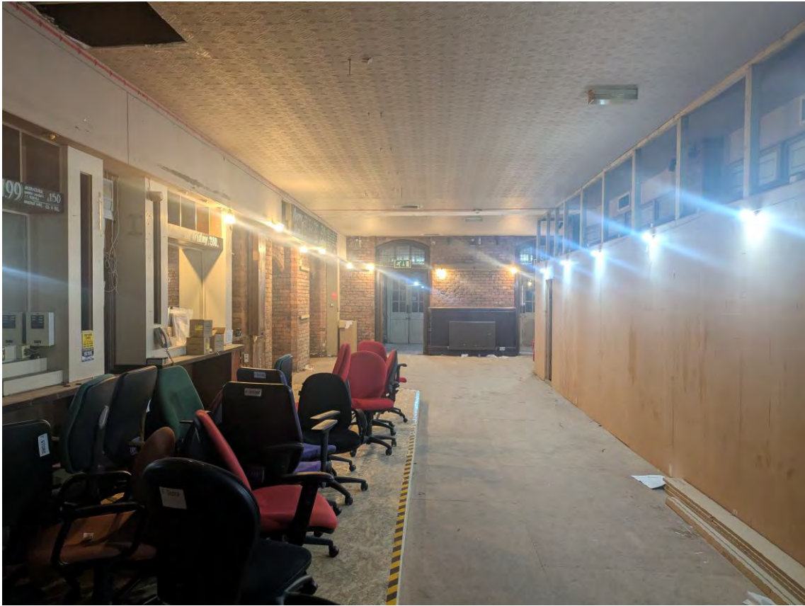
Plate 8: 20th Century Disruption to Internal Fabric and Entrance
