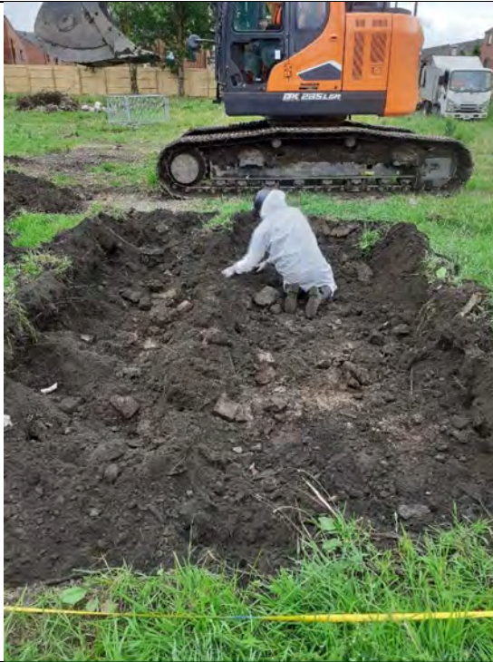
Figure 3: Close search through excavated shallow soils for ACM within contaminated area
