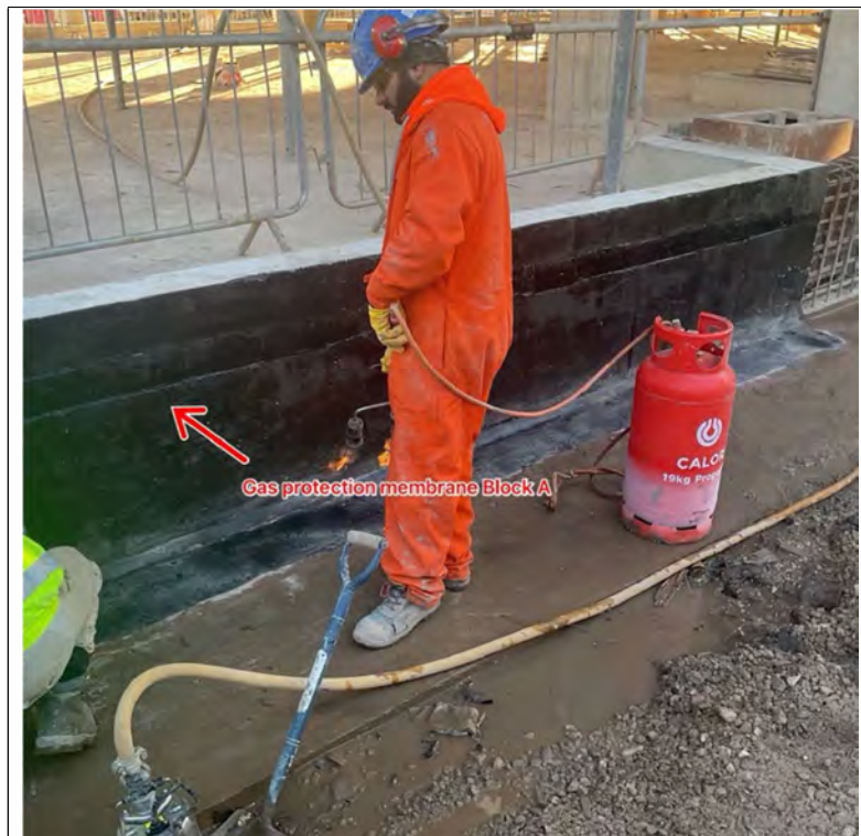
Figure 8: Sealing of gas protection membrane to Block A
