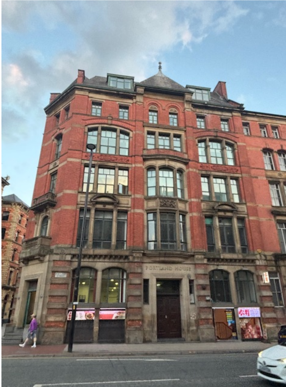
1.2.4 North Elevation. Portland Street.
