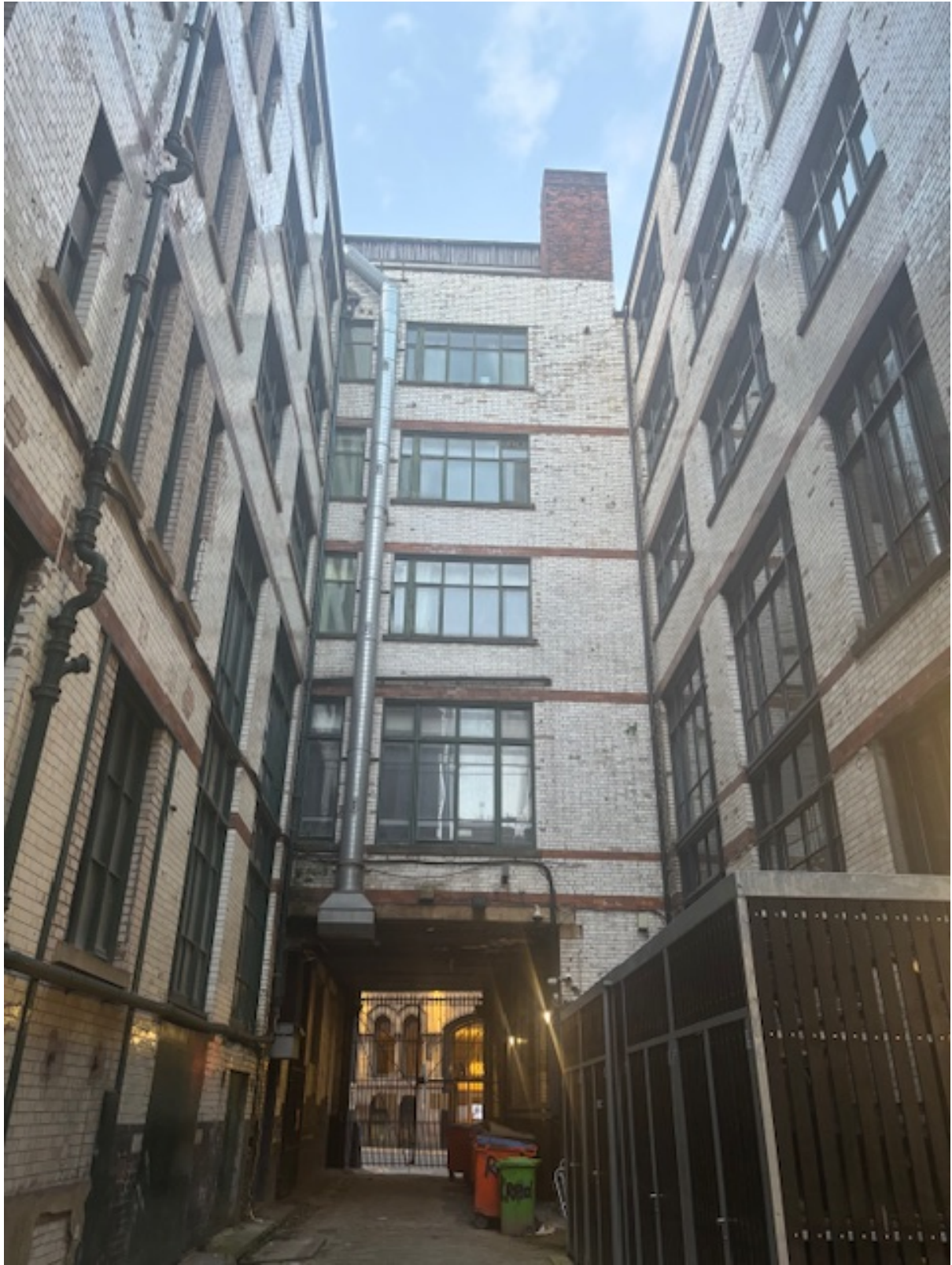
1.2.6 Rear Elevation Courtyard. Showing Undercroft.
