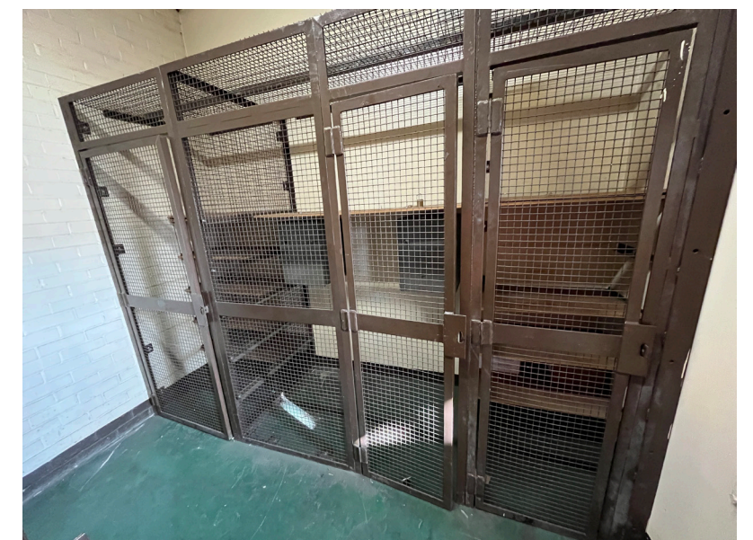
GF.08 Vault cages
