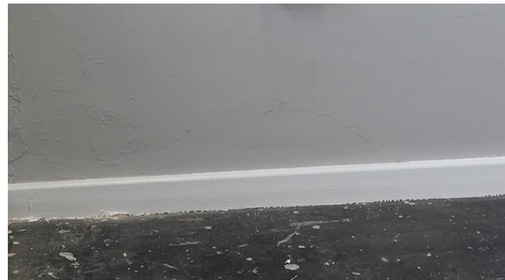
Example of existing skirting
