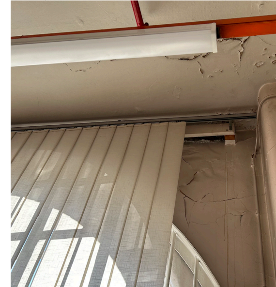
Blinds fixed above arched windows obscuring the form will be removed. New blinds are proposed which follow the curve of the arch and are secret fixed within the window reveal.
