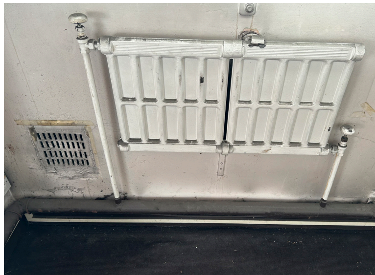
Radiators to be retained
