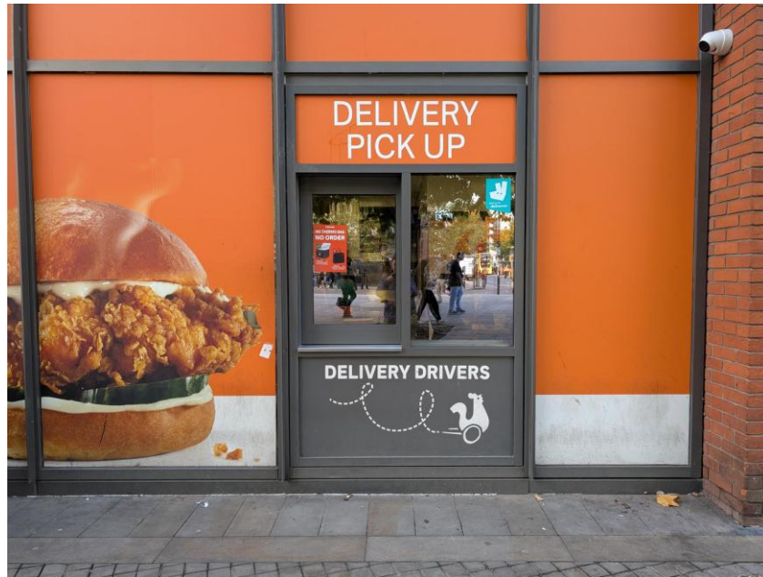
Figure 1: Existing service hatch installed prior to the refusal of application 137200/FO/2023, photo taken 06/10/2025.
