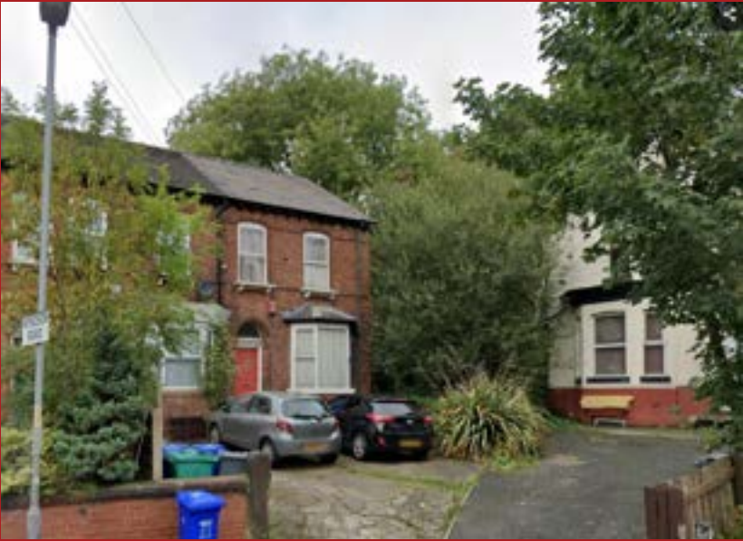
The Existing Building On Site
