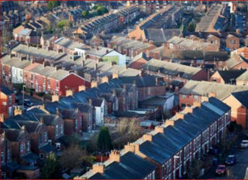
Aerial view of Levenshulme Streets
