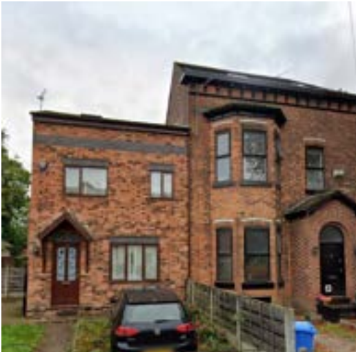
Windsor Road - modern brick (extension) with vertically stacked grey detailing
