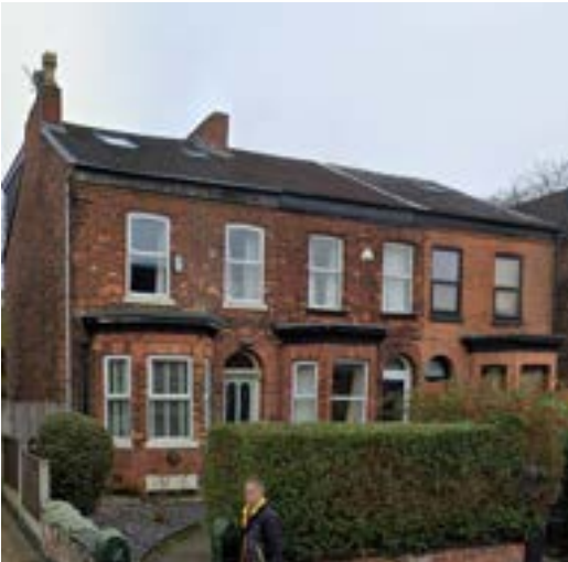
Buckhurst Road - dark red/brown brick with black detailing
