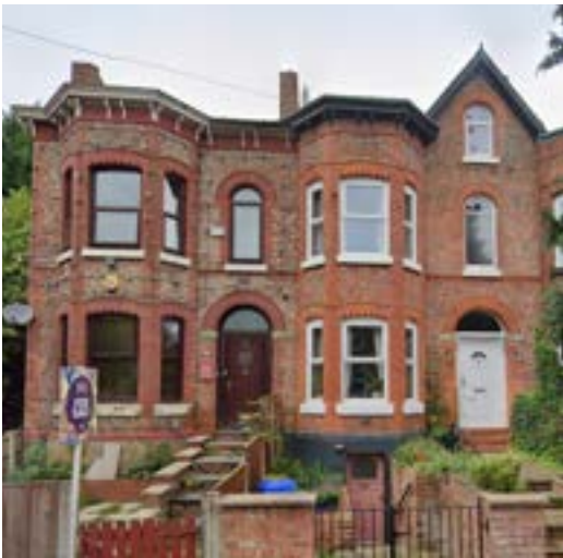
Osborne Road - brown brick with buff and red brick traditional detailing
