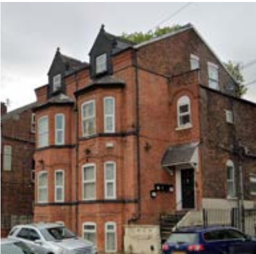
Osborne Road - red brick with black detailing
