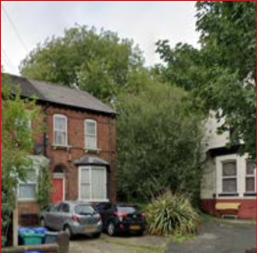
Front elevation of the existing house
