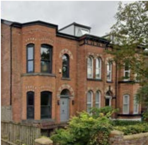
Windsor Road - red brick with buff brick traditional detailing
