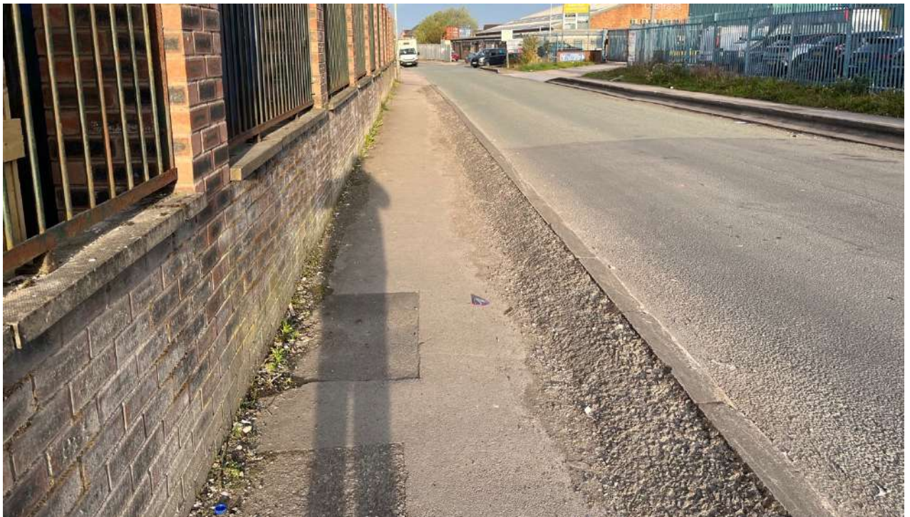
Photograph 3.3 : Station Road – Footway Provision
