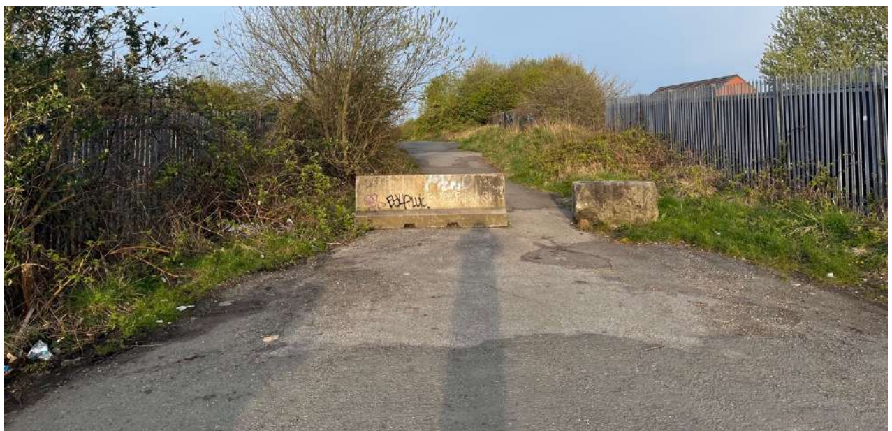
Photograph 3.5 : Existing Site Access and Bridge
