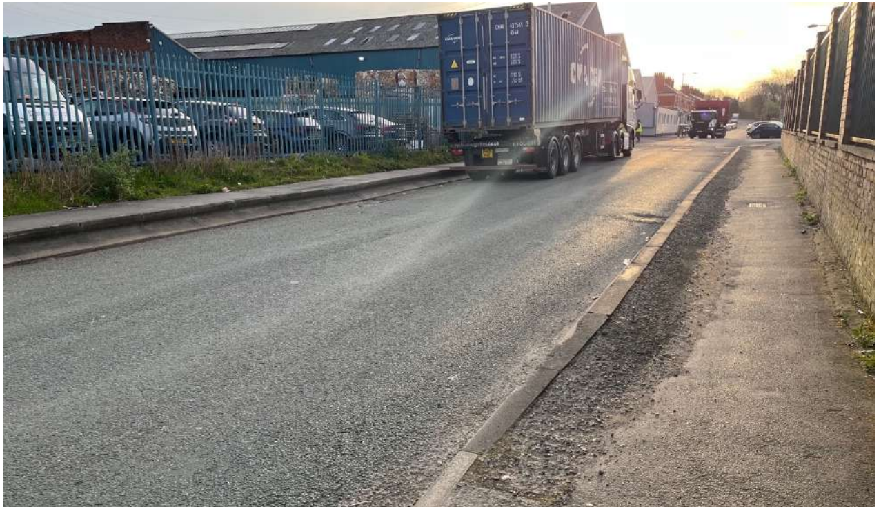
Photograph 3.2 : Station Road – Titan Kerbs
