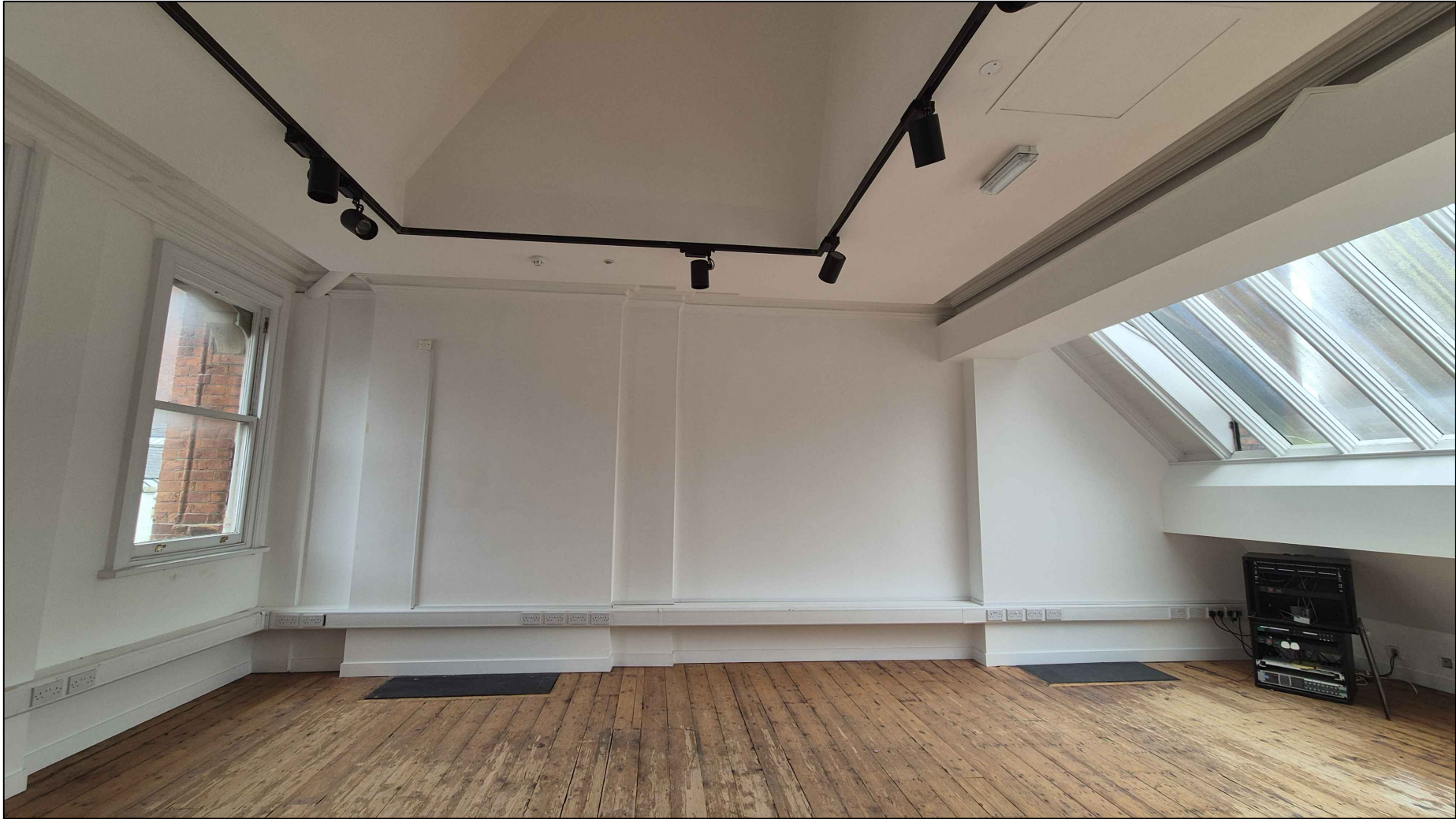
3rd Floor - EXISTING - photo
