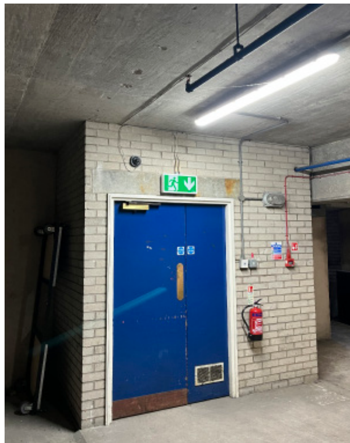
Figure 4 Basement, the basement contains exposed concrete soffits and brickwork walls. The doors and frames are later addition insertions, existing fixing points will be re-used with new screw and plug fixings wherever possible to reduce the impact of the installation.
