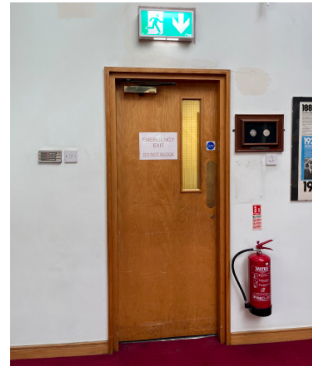
Figure 15 Typical Door to be Upgraded, oak veneer doors with Doc M compliant vision panels and brass ironmongery compliment the existing spaces.
