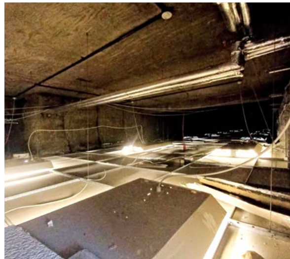
Existing ceiling void condition lacking features
