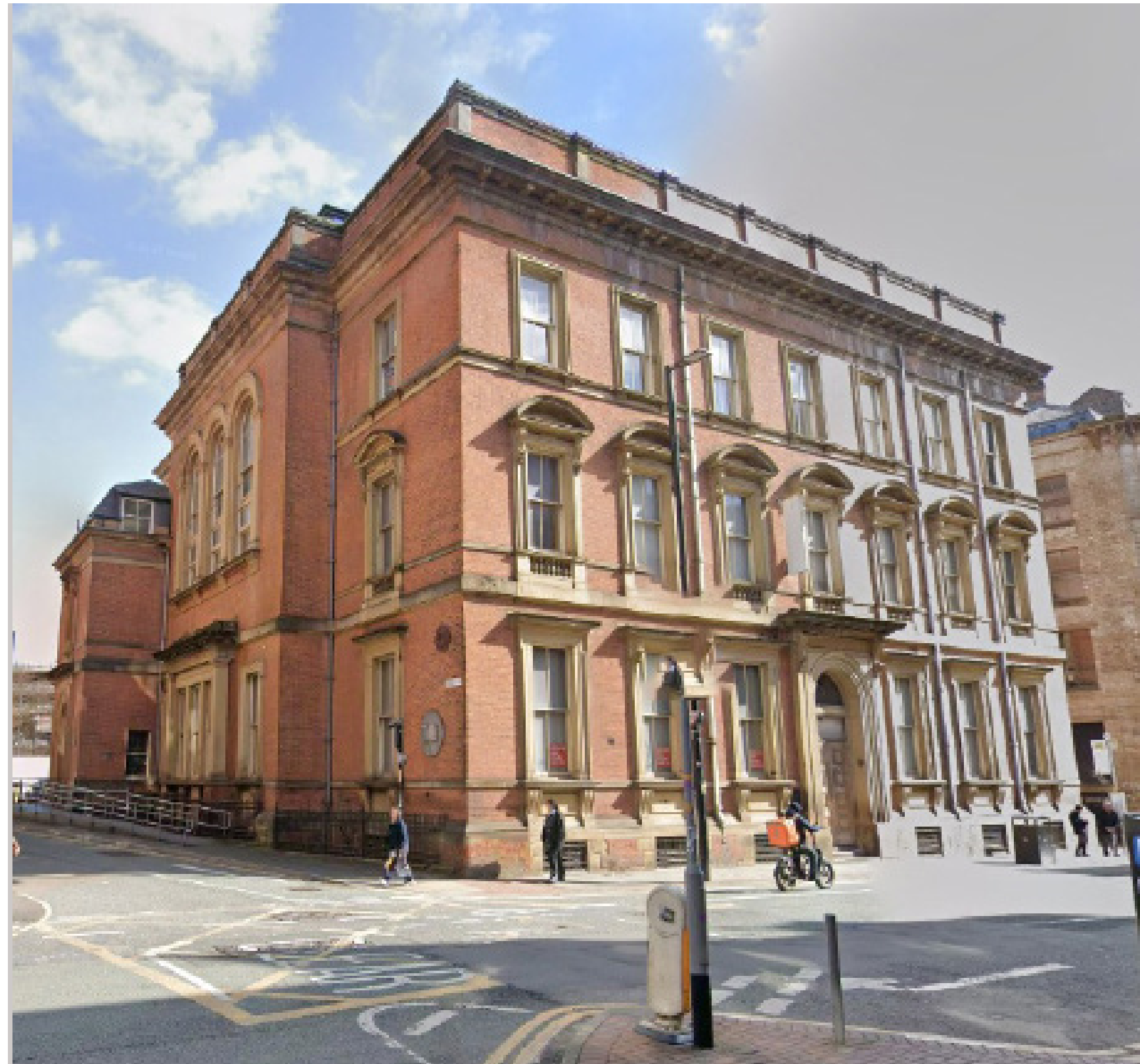
Figure 3 103 Princess St from junction of Harter St and Princess St
