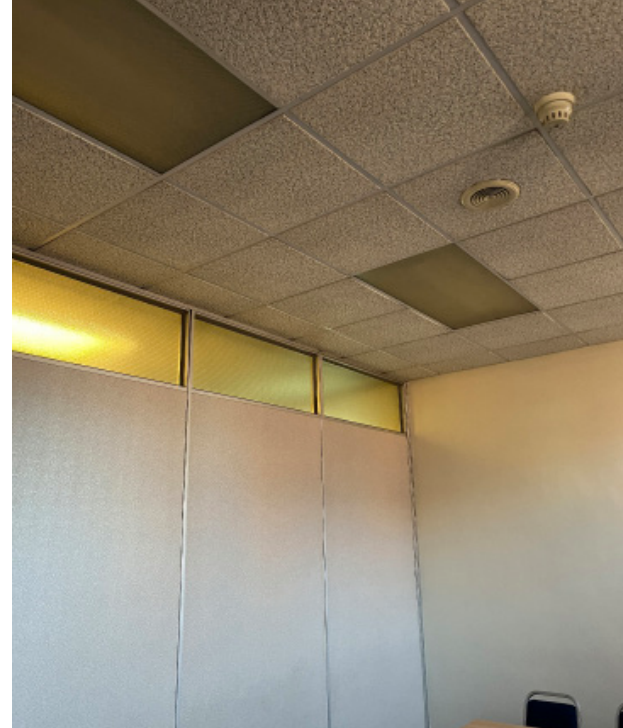
Figure 13 Level 03 Alcove Room, wireless fire detection equipment re-using existing positions is proposed to these areas with higher historic significance.
