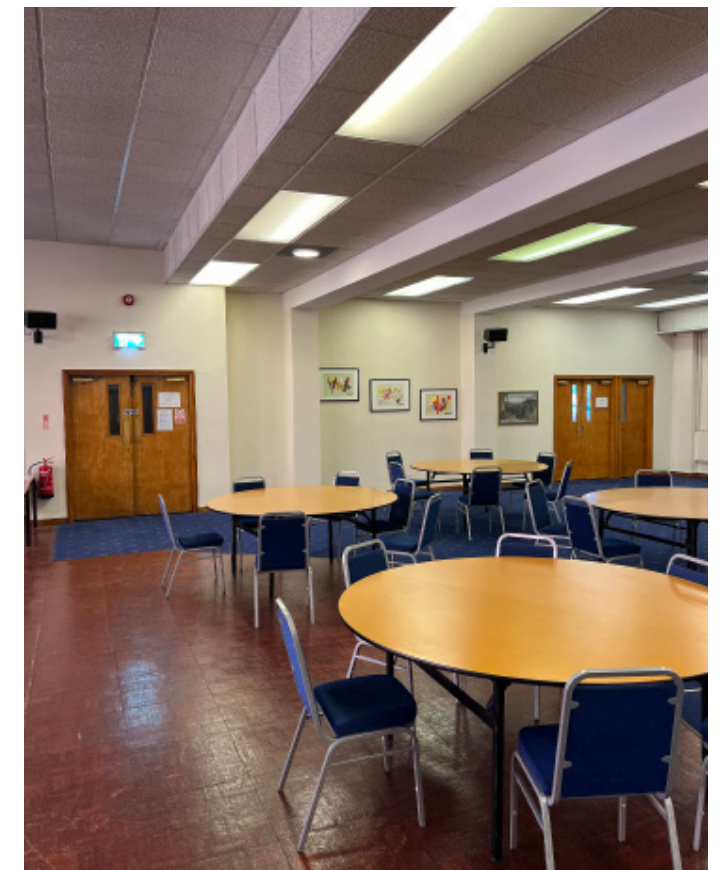
Figure 7 Level 012 Main Hall, these areas have later addition suspended ceilings present which are to be retained. The fire alarm installation will be on a like-for-like basis with new sounders and detector heads.
