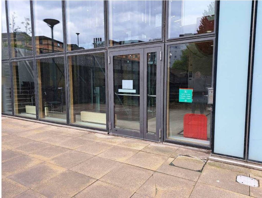
Photo 3: Existing manual fire escape door at lower ground floor level, adjacent to the passenger lifts.
