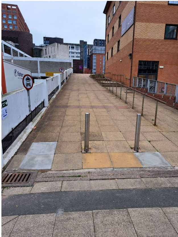
Photograph 2: Ramped and stepped access from Sackville Street towards the main entrance of John Garside Building.
