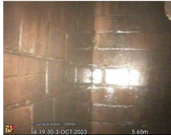
MH4A DS MH5_5-65m_141930.jpg, 00:00:33, 5.65 m Finish node, manhole, reference: MH5, CULVERT MH
