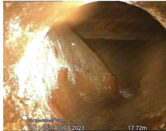
MH24 DS_17-72m_101457.jpg, 00:01:15, 17.72 m Finish node, manhole, reference: DS, UNCHARTED, POSS UNDER CABINS
