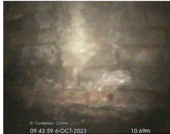
MH C1 DS_10-69m_094359.jpg, 00:00:47, 10.69 m Finish node, major connection without manhole, reference: DS, CULVERT
