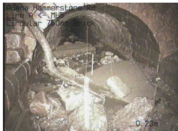
Line AX_8e7aa481-461d-44bb-8f15-7b653cb4fe82_20230928_100 930_894.jpg, 00:00:24, 0.23 m General remark, General MH survey
