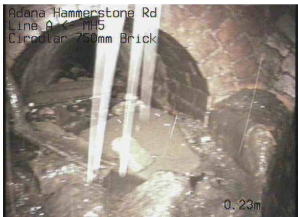
Line AX_e91a9475-7b4e-47fb-a422-8ee038e079f9_20230928_100 927_614.jpg, 00:00:24, 0.23 m General remark, General MH survey
