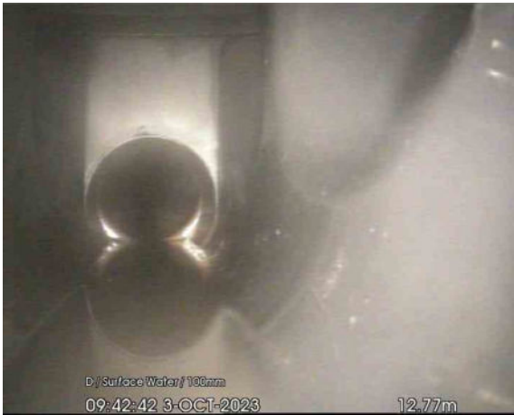
MH17 DS MH18_12-77m_094242.jpg, 00:00:47, 12.77 m Finish node, inspection chamber, reference: MH18, DIP IN CHAMBER
