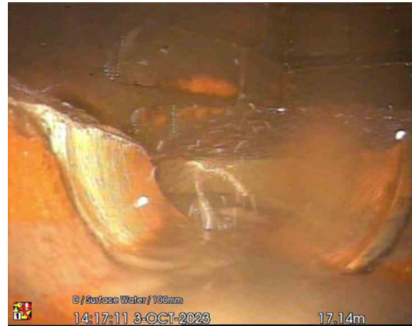
MH4 DS MH5_17-14m_141711.jpg, 00:02:08, 17.14 m Finish node, manhole, reference: MH4A, UNCHARTED MH
