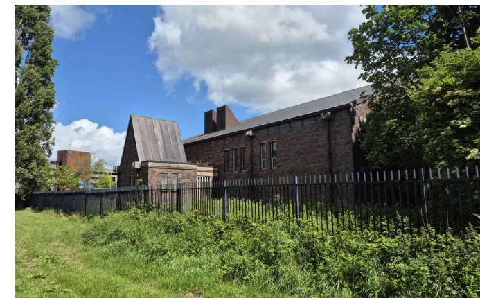
Relevant Area View from South
