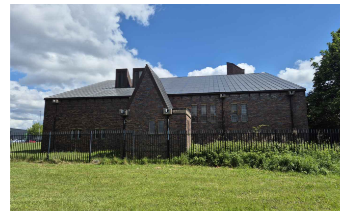
Relevant Area View from South-West
