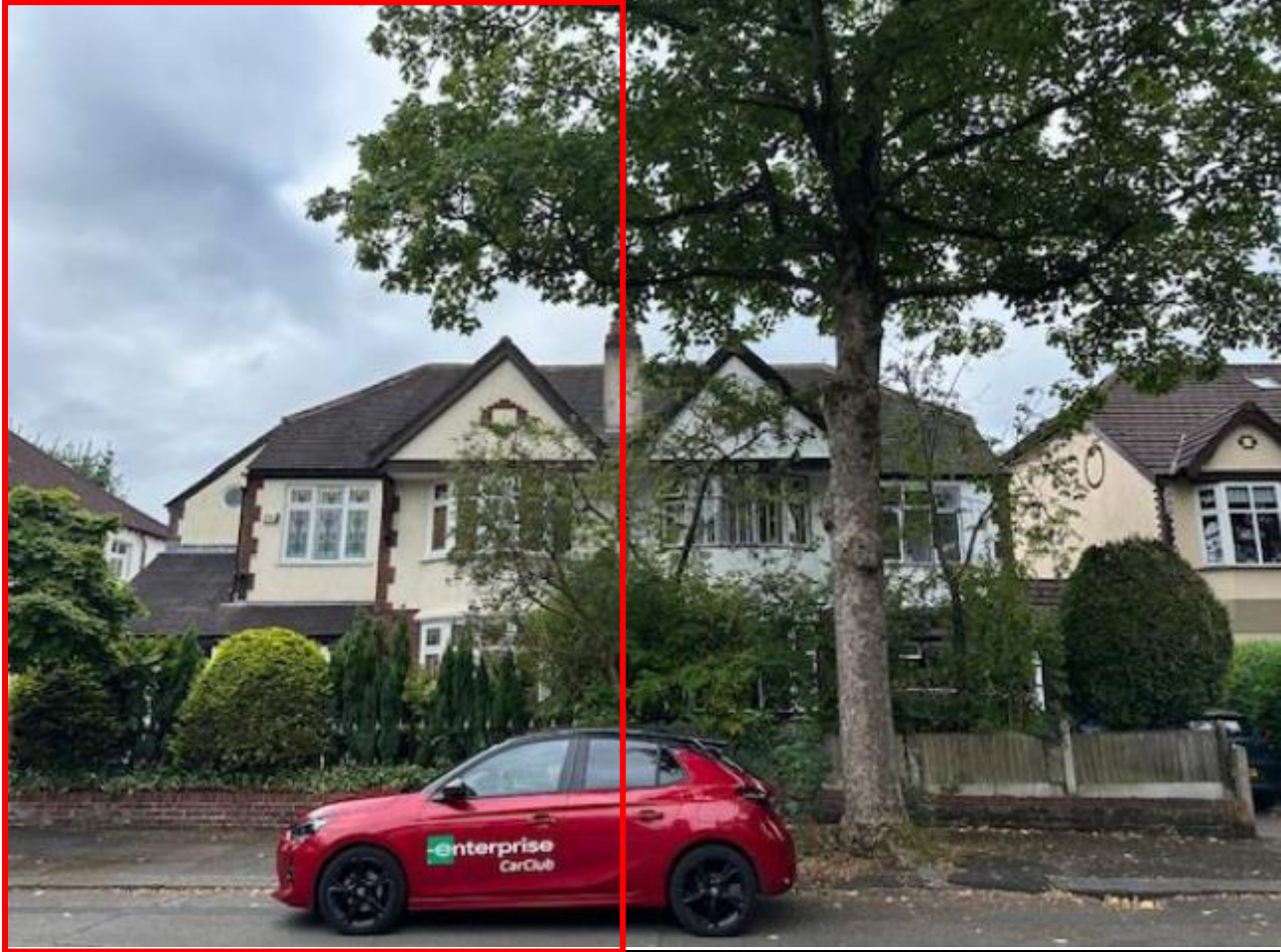
Figure.1 The application property, no.9 and the adjoining semi, no.11.
