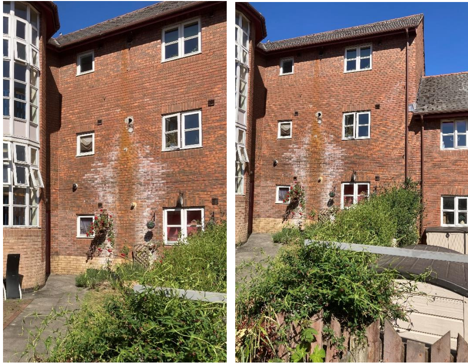
Flats 1-9, 2 Jackson Crescent - Rear Elevation (View G)
