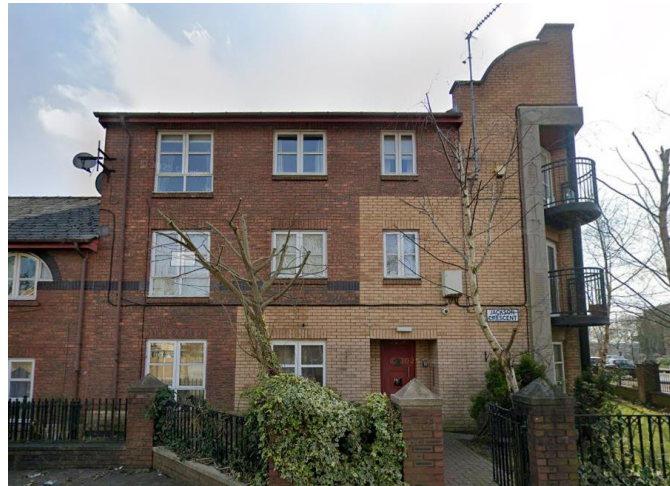
10, 12, 14, 16, 18, 20 Jackson Crescent & Flats 1-9, 2 Jackson Crescent – Front Elevation (View C)
