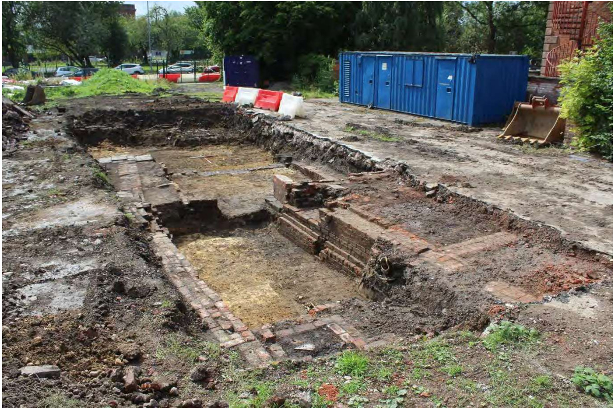
Plate 17: General view of the initial exposure of the north-eastern end of the excavation area showing the remnants of walls associated with the Sunday School and outbuilding
