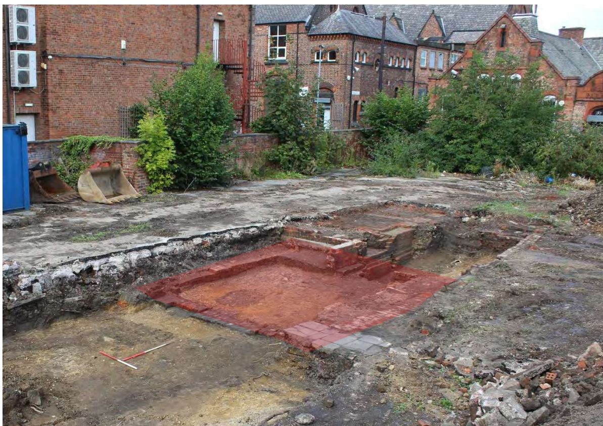
Plate 15: General view looking north across the footprint of the single-depth house, highlighted red
