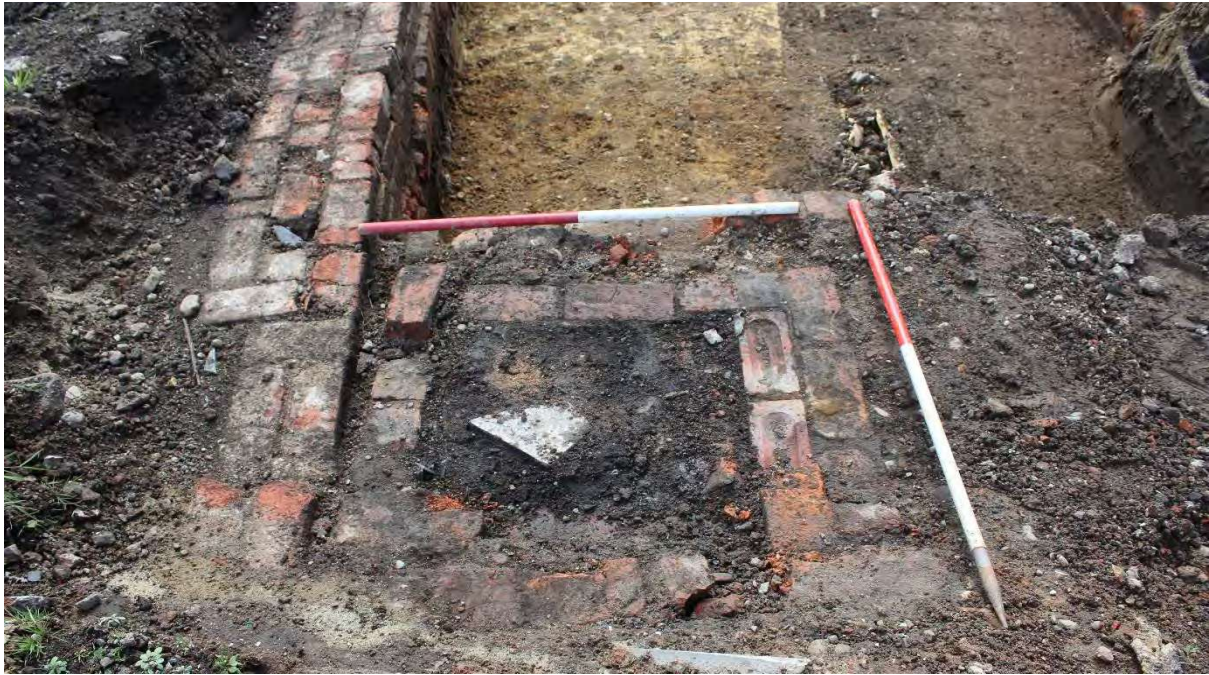
Plate 22: Brick manhole [023]/[024]/[025] looking south-west (scales: 1m)
