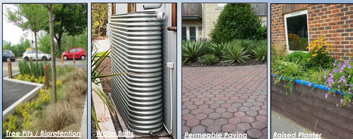
Figure 3: SuDS Photographs (SusDrain, 2012)
